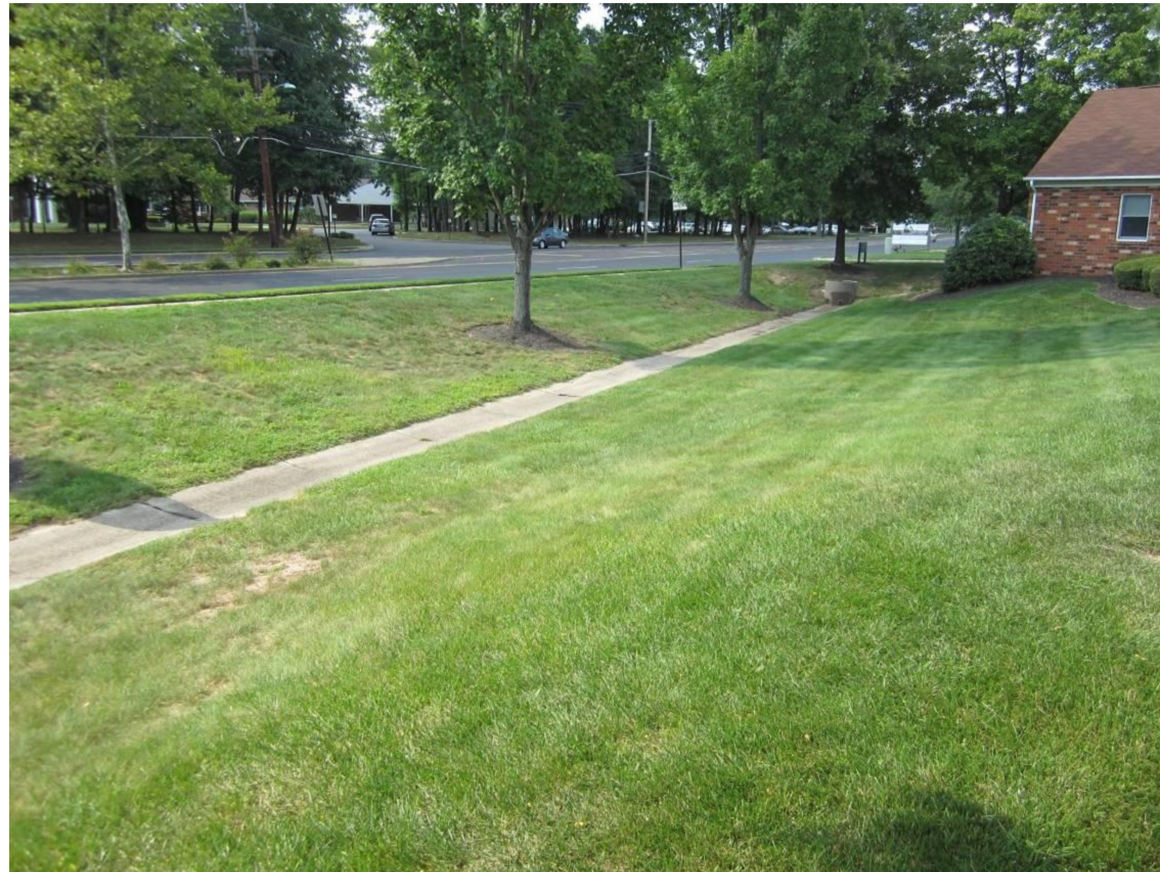
Basin bottom looking north
