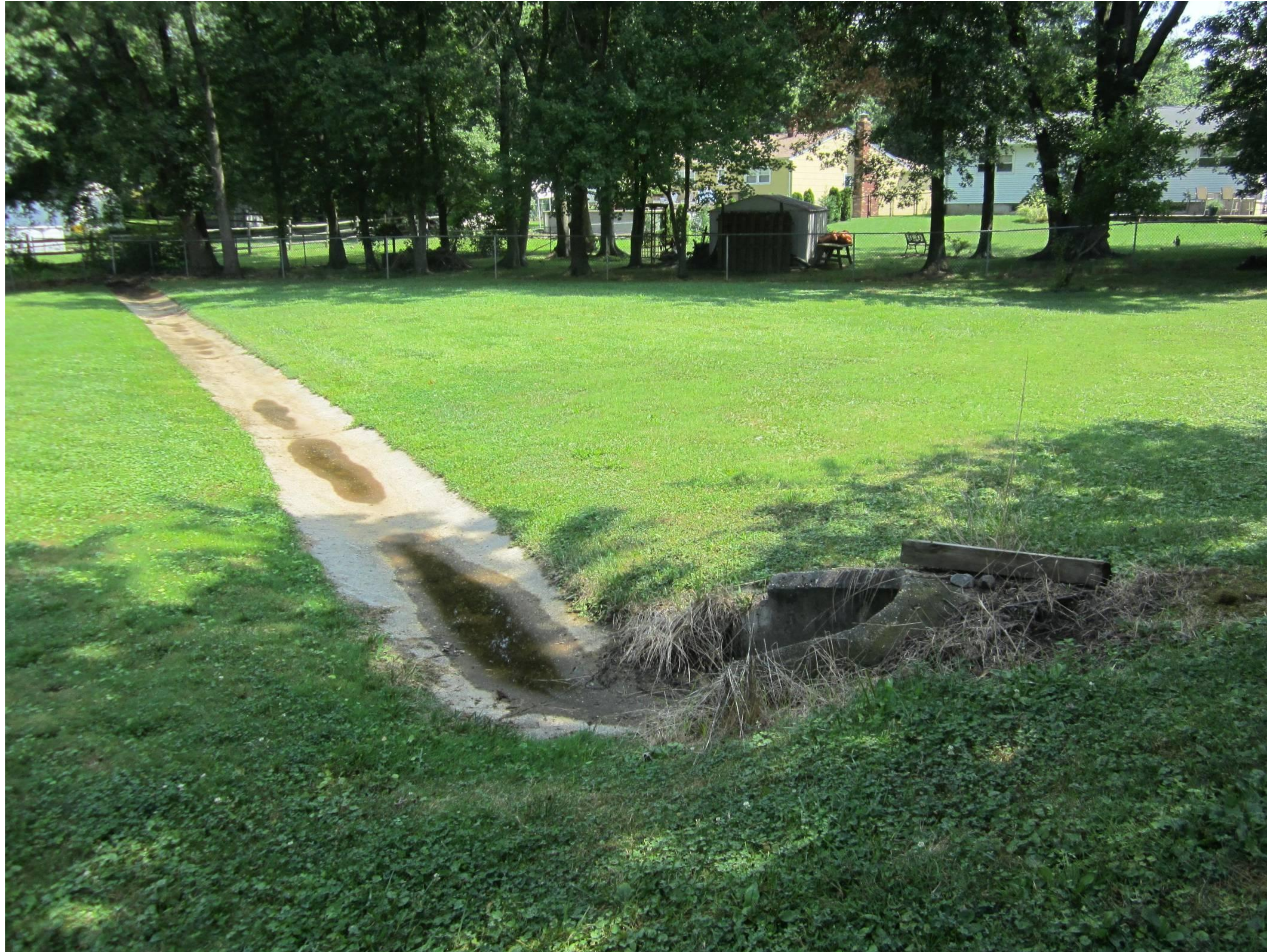
Entire Basin looking northeast
