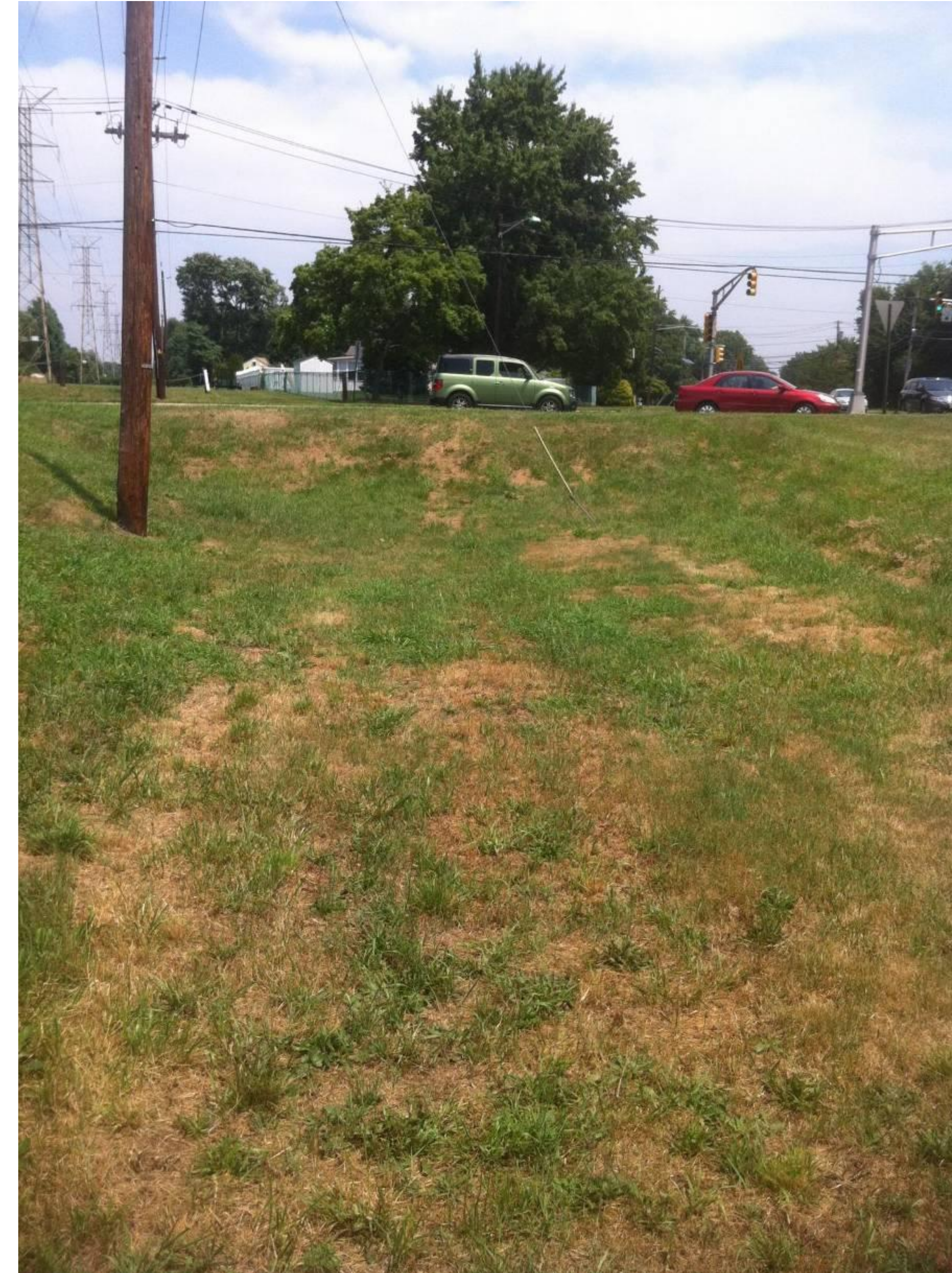
Basin bottom looking east
