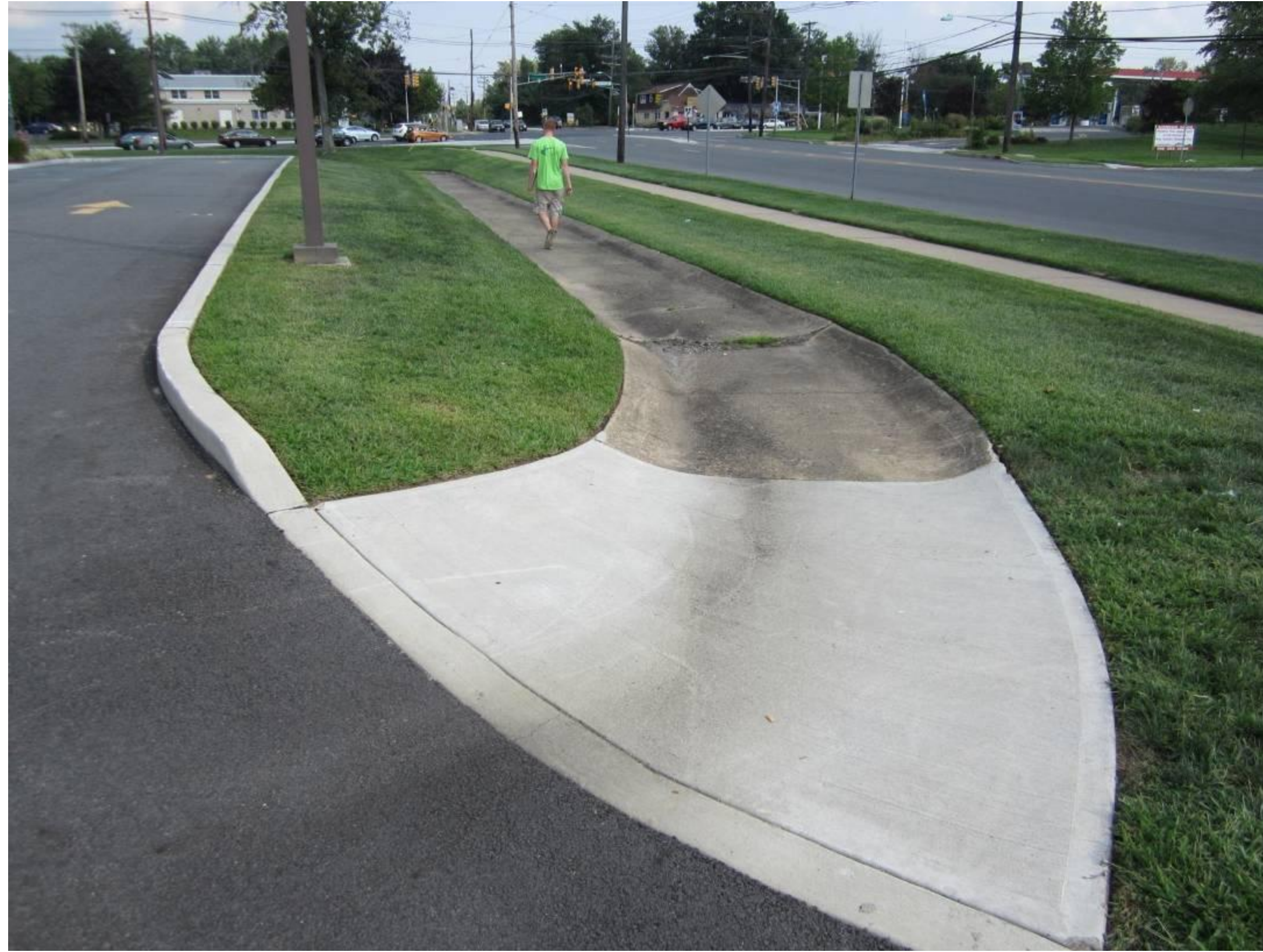
Inlet curb cut
