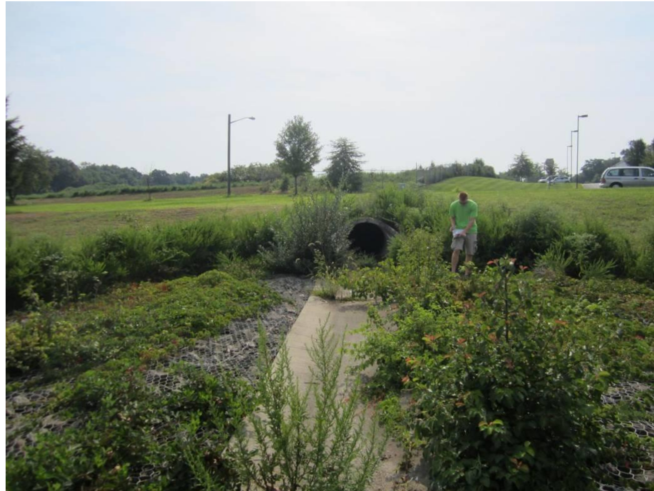
Inlet and rip rap protection
