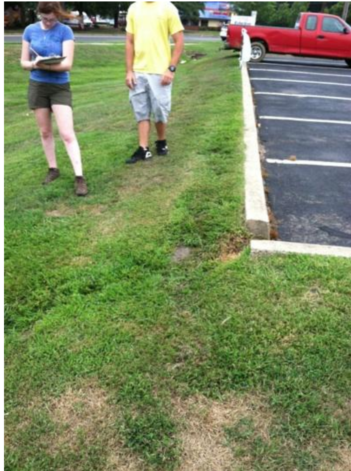
Erosion at inlet
