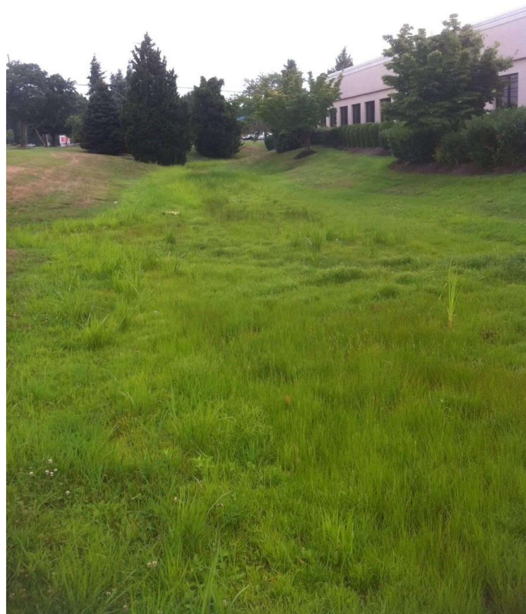
Basin bottom looking northeast
