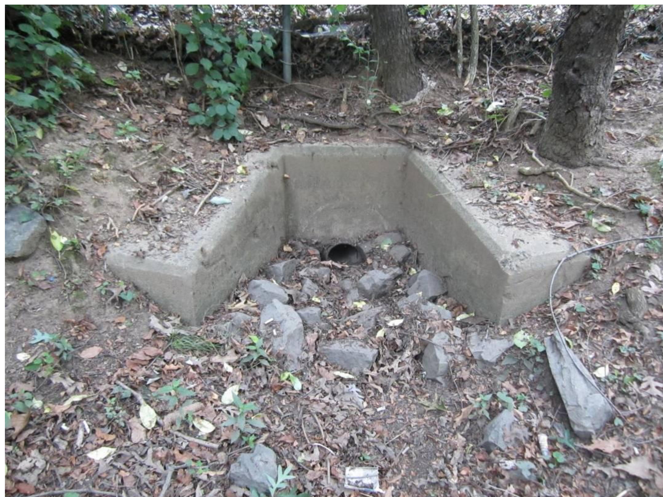
Outlet with woody vegetation and sediment
