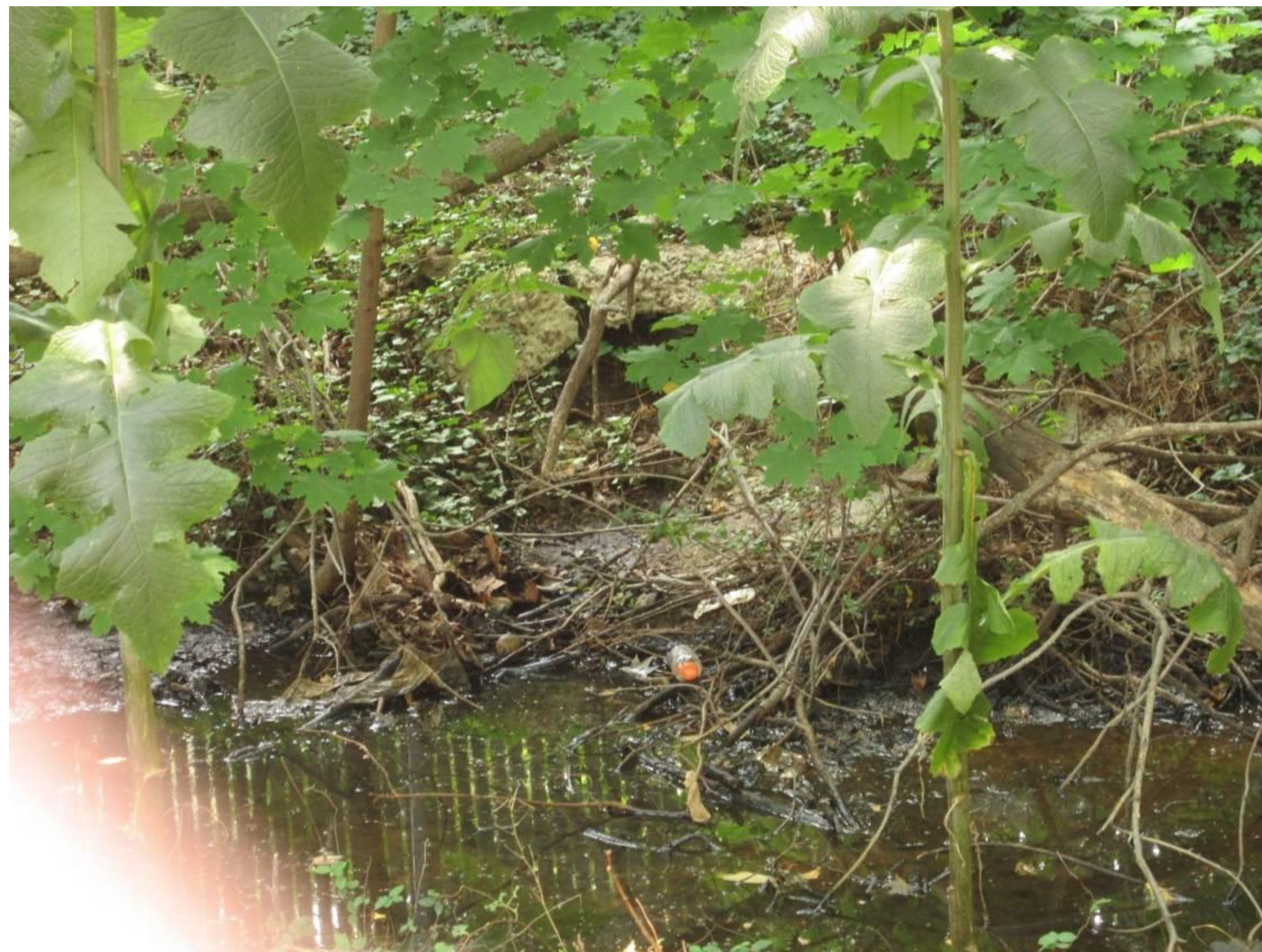
Ponding in basin bottom
