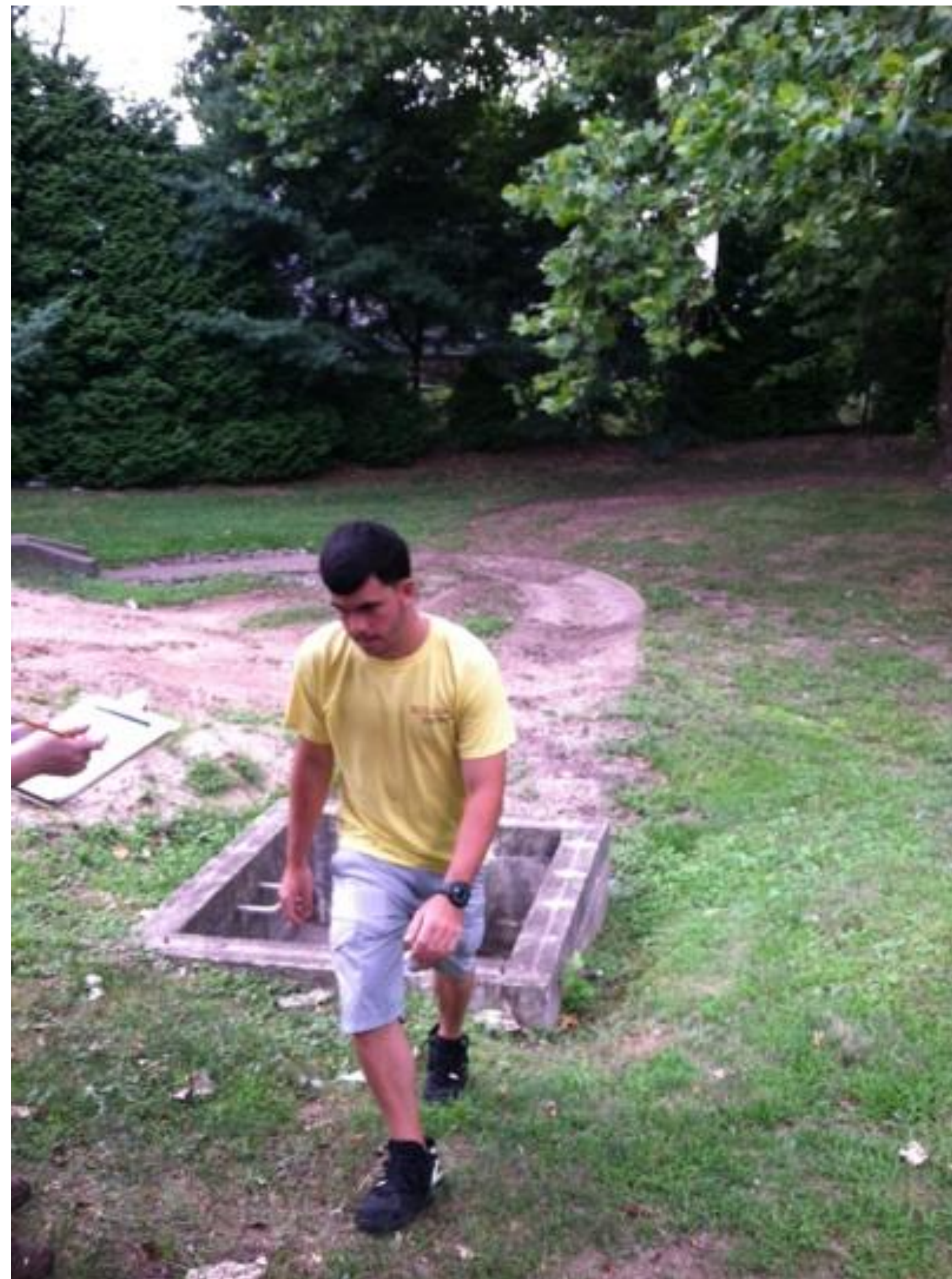
View of basin looking east
