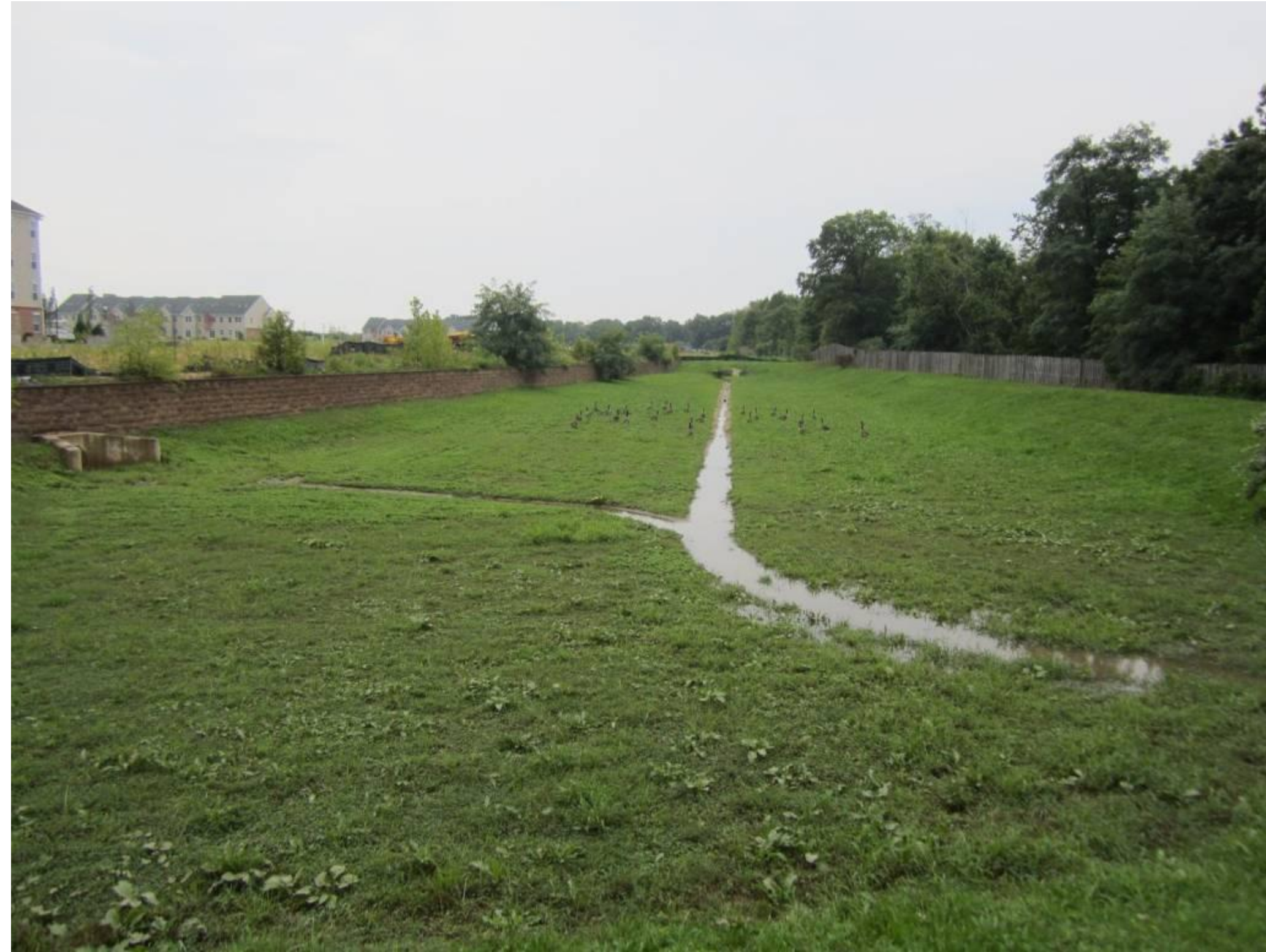
Basin bottom looking southwest
