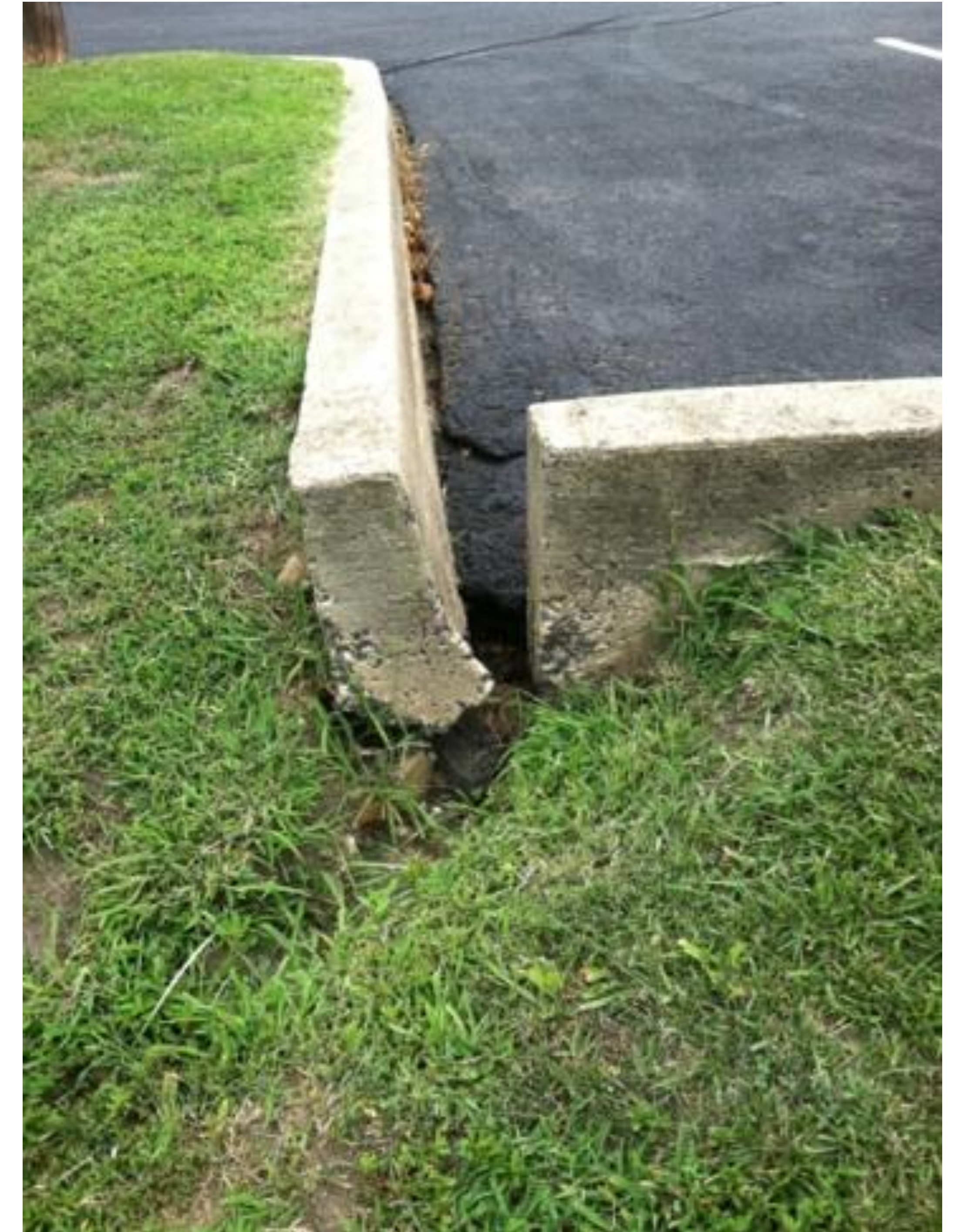
Damaged inlet
