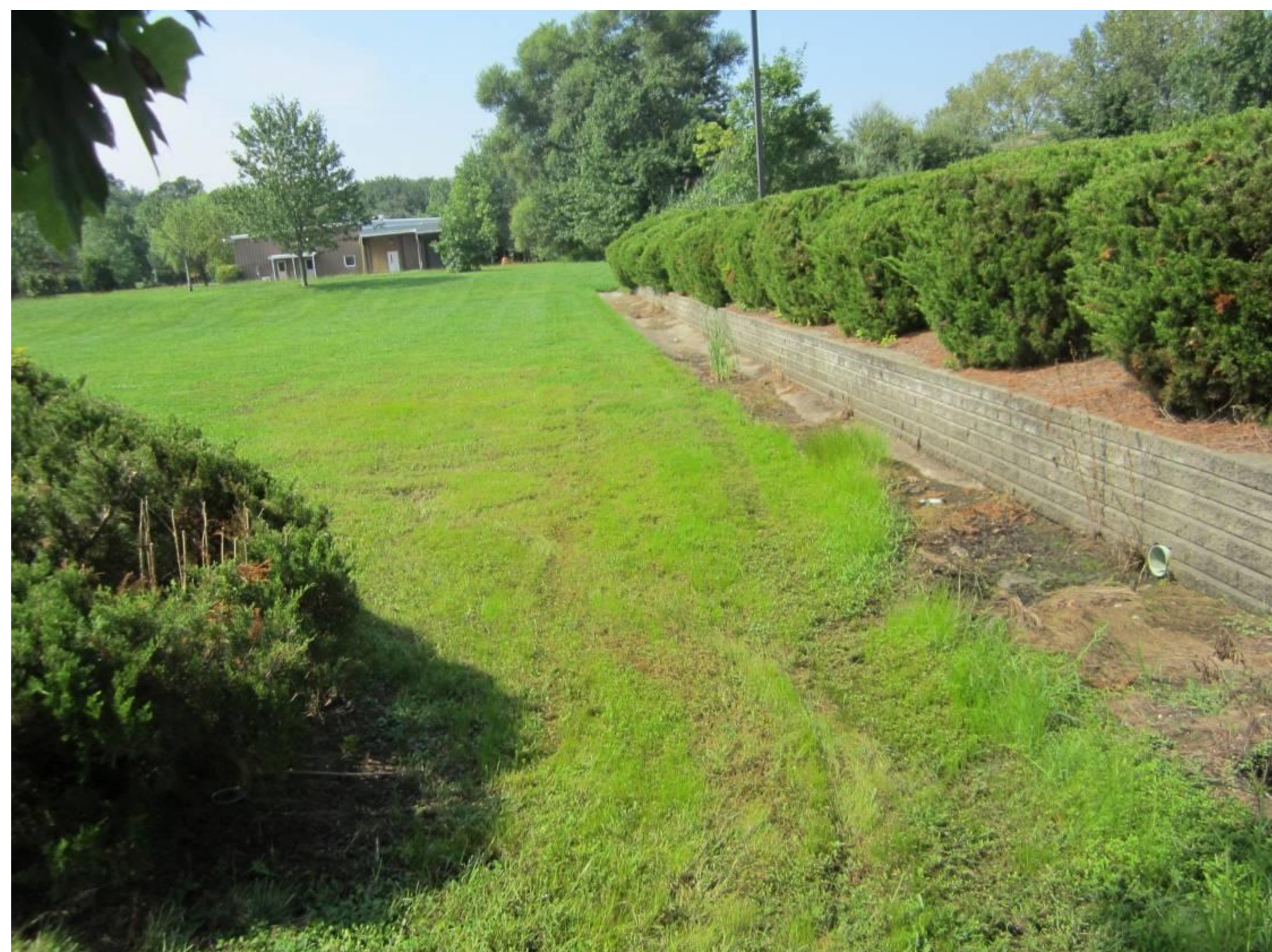
Basin bottom looking northeast
