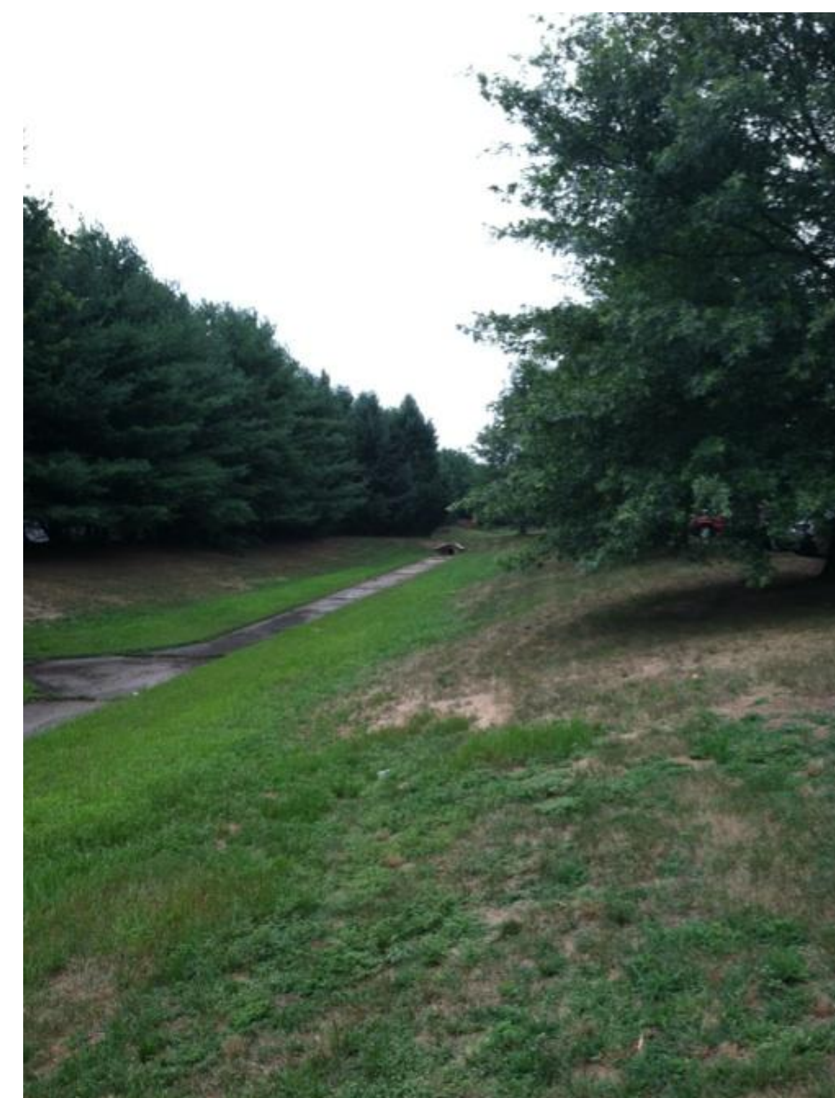
Basin bottom looking southwest
