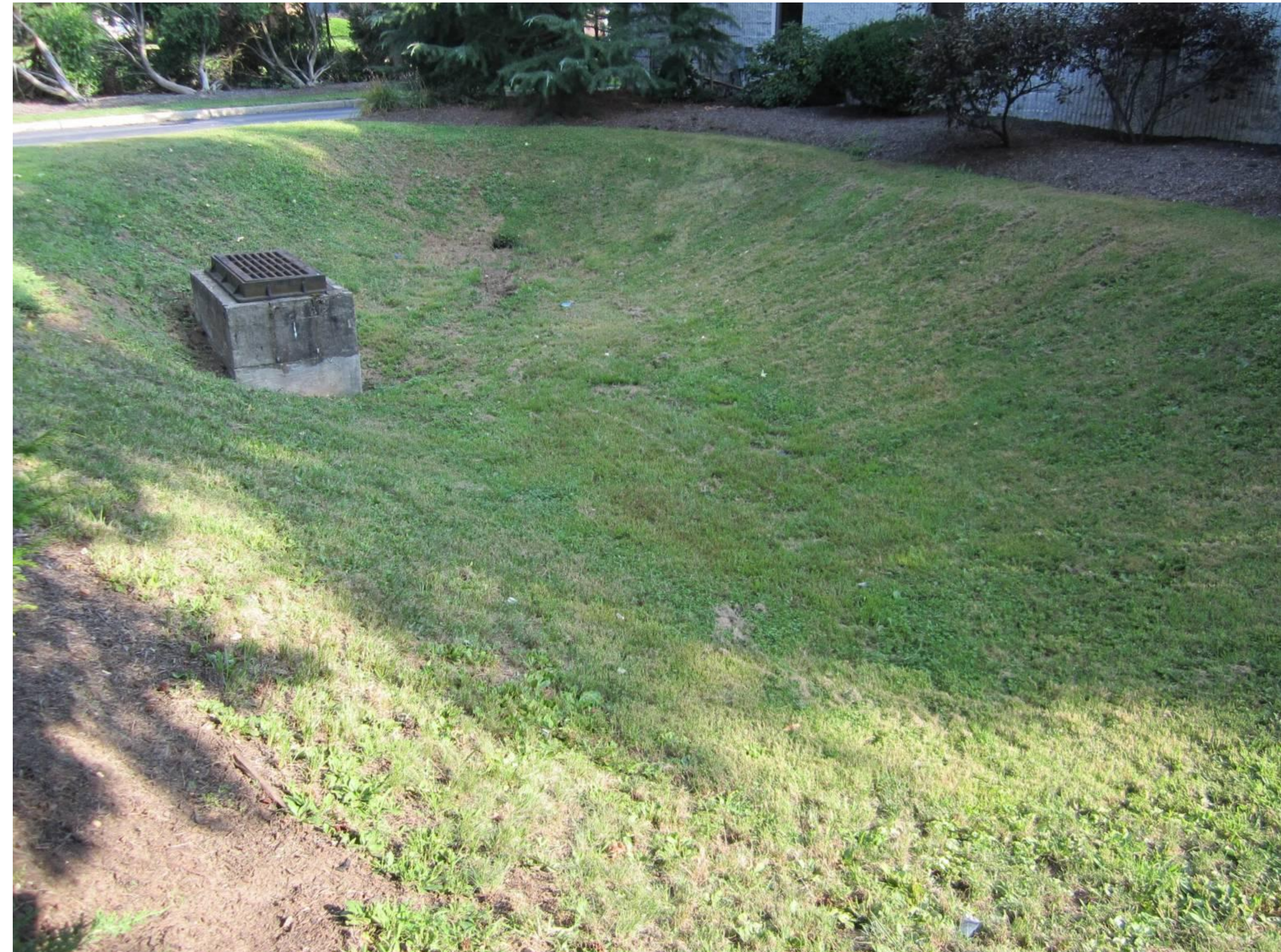
Basin bottom looking east
