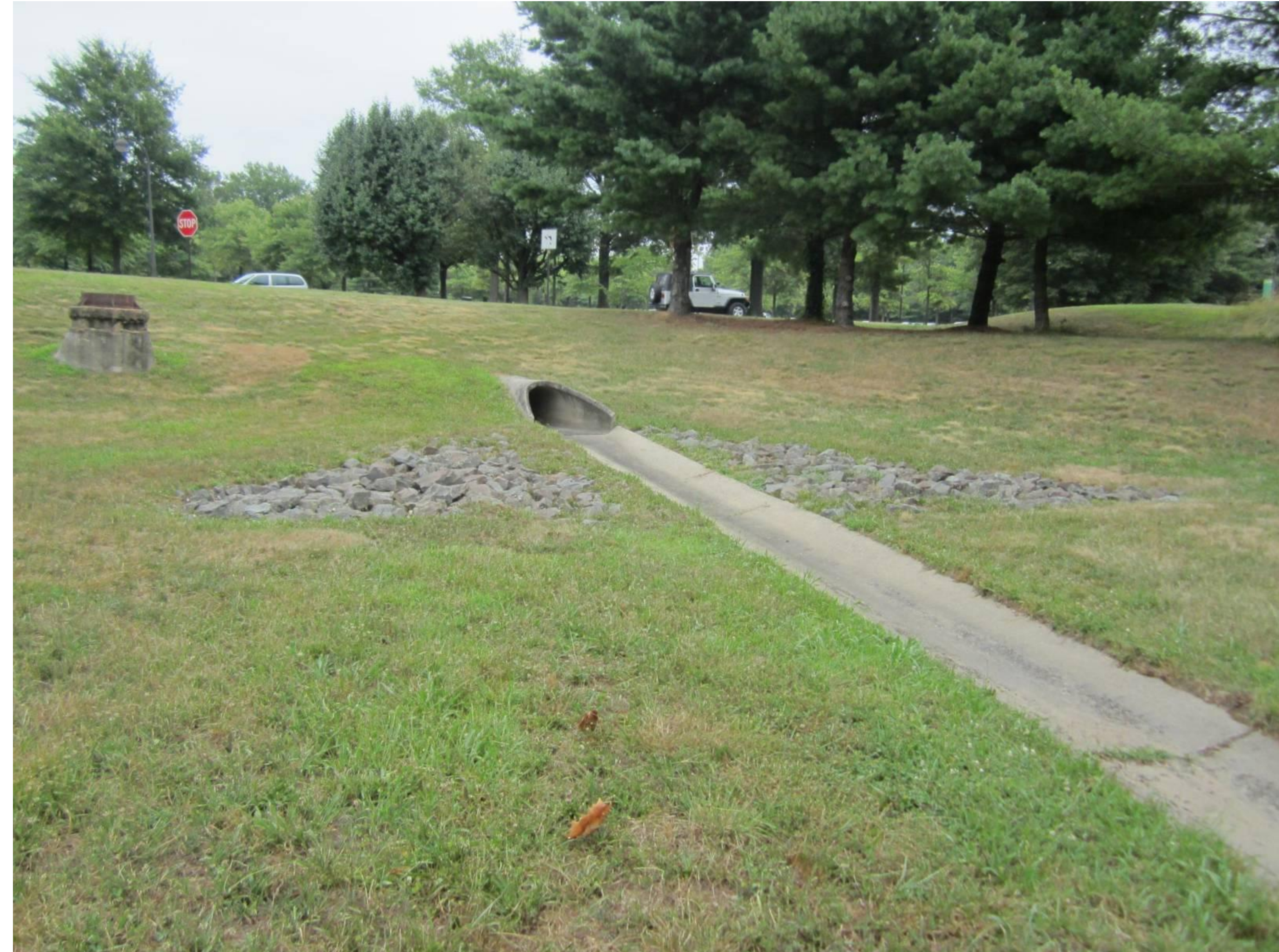
Inlet and rip rap
