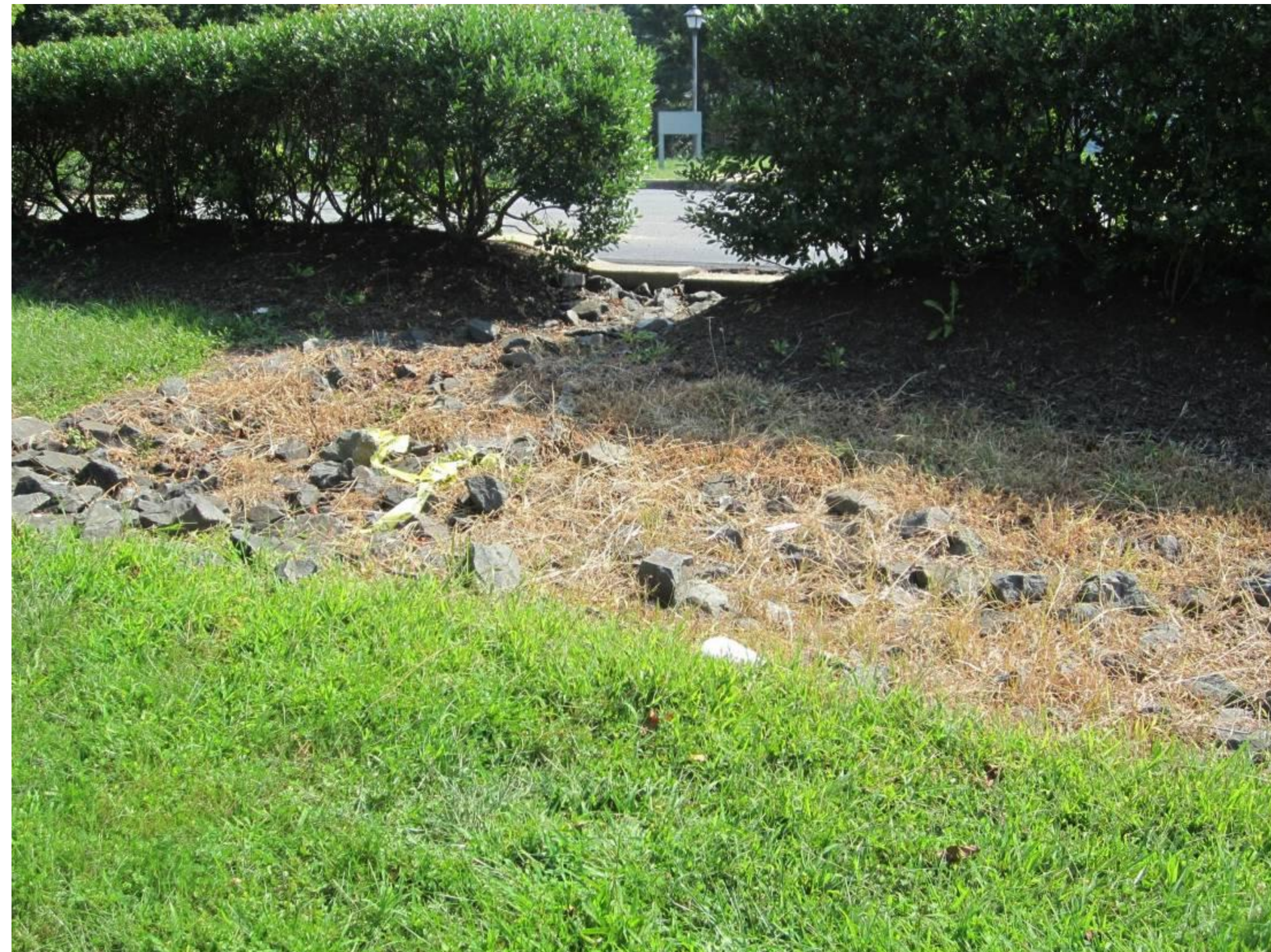
Curb cut inlet with rip rap protection
