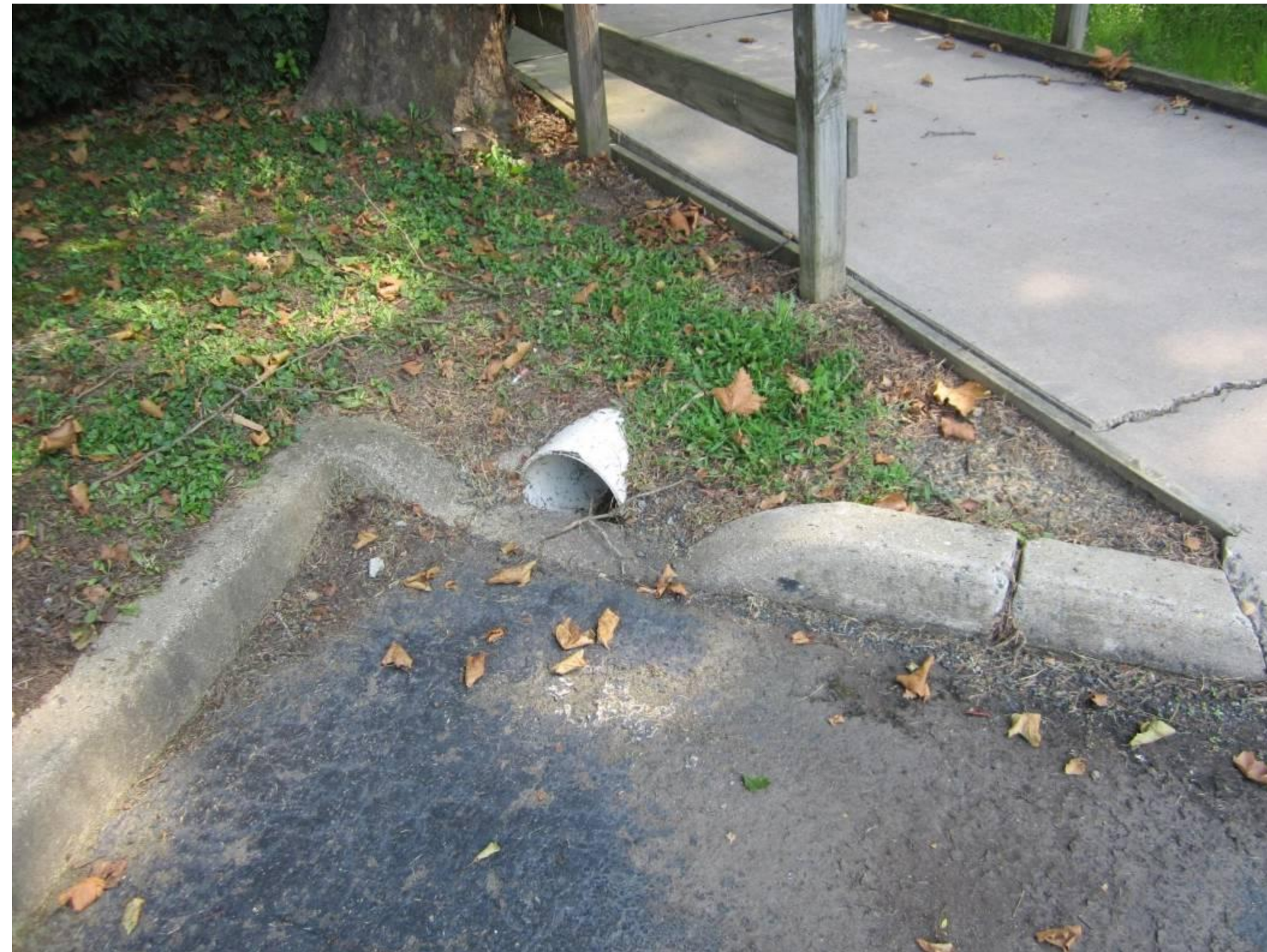
Curb cut with PVC pipe
