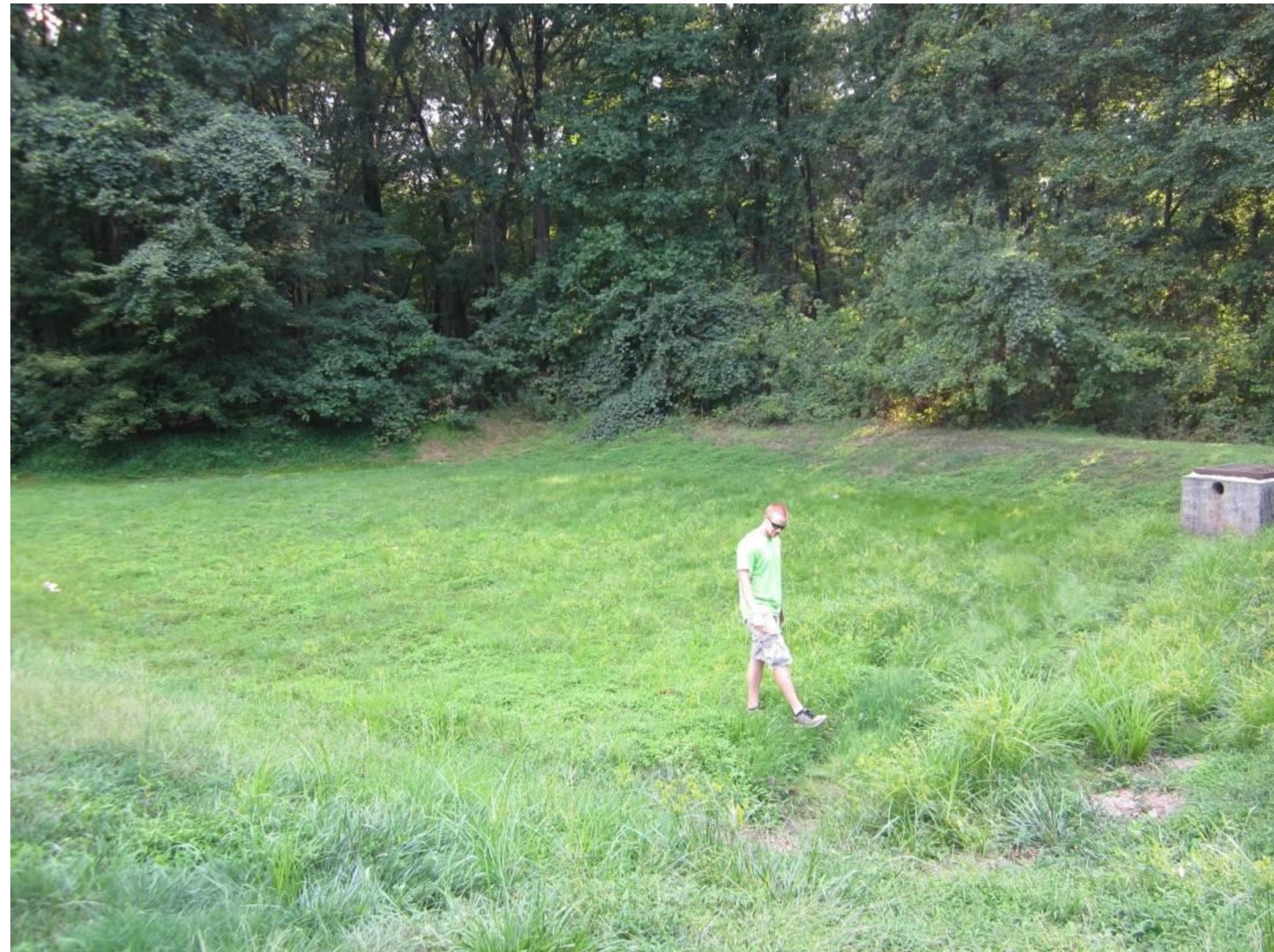
Basin bottom looking northwest
