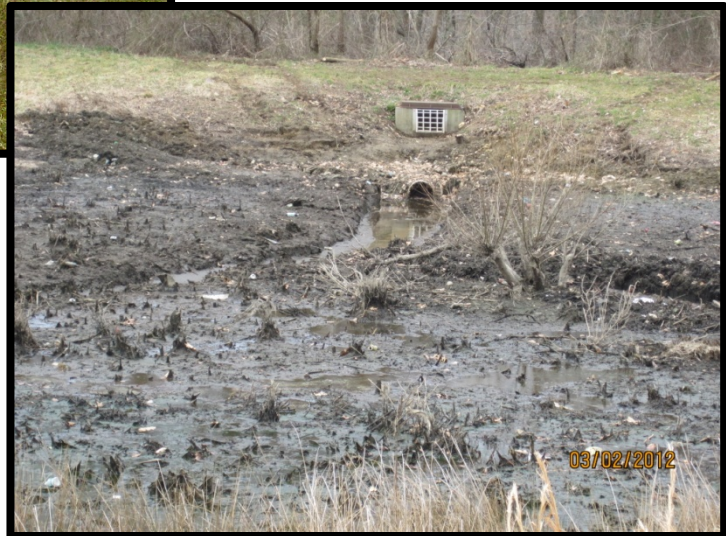
Kristopher Drive Basin After Cleaning (2012)
