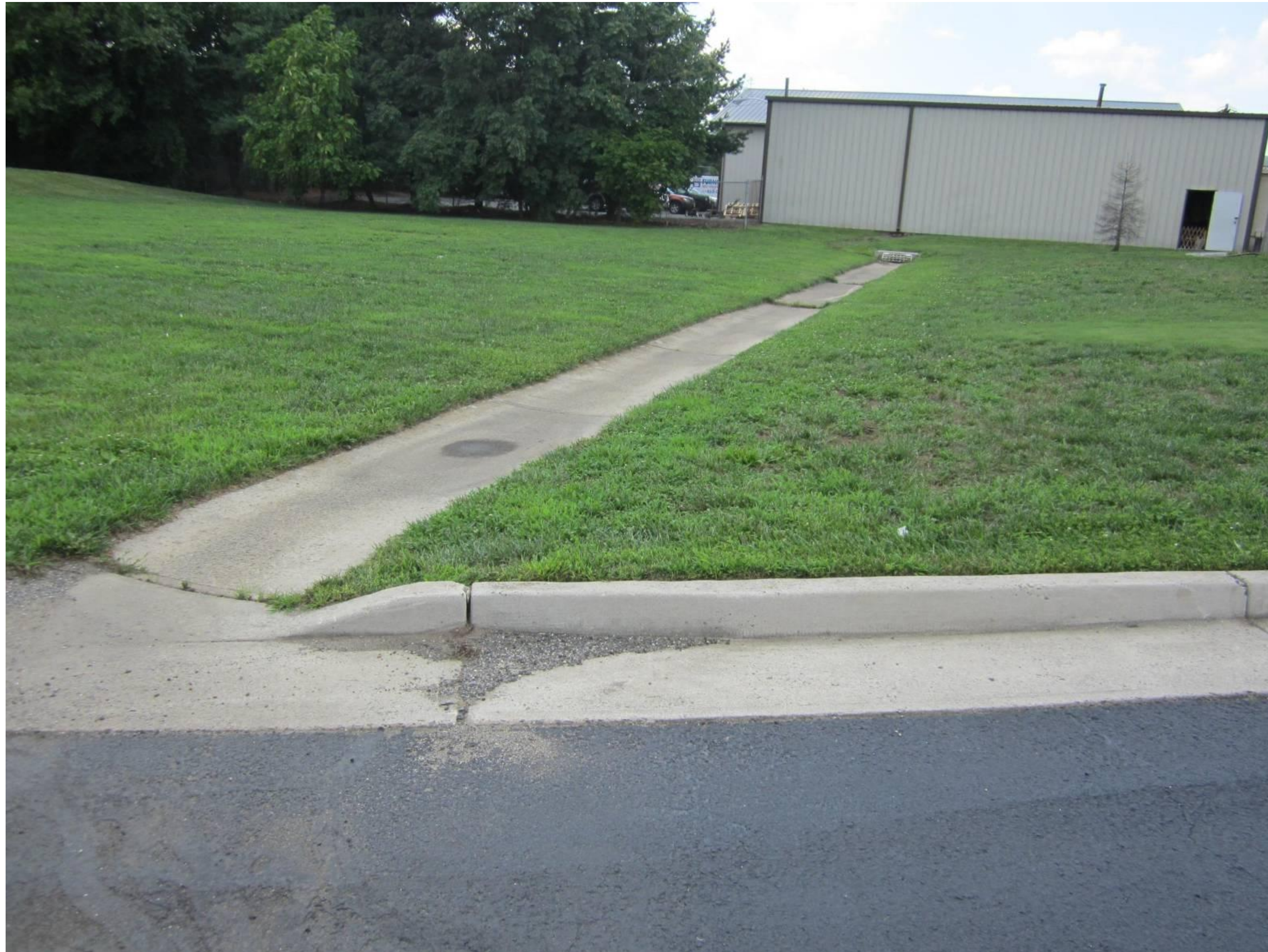
Curb cut inlet and low flow channel
