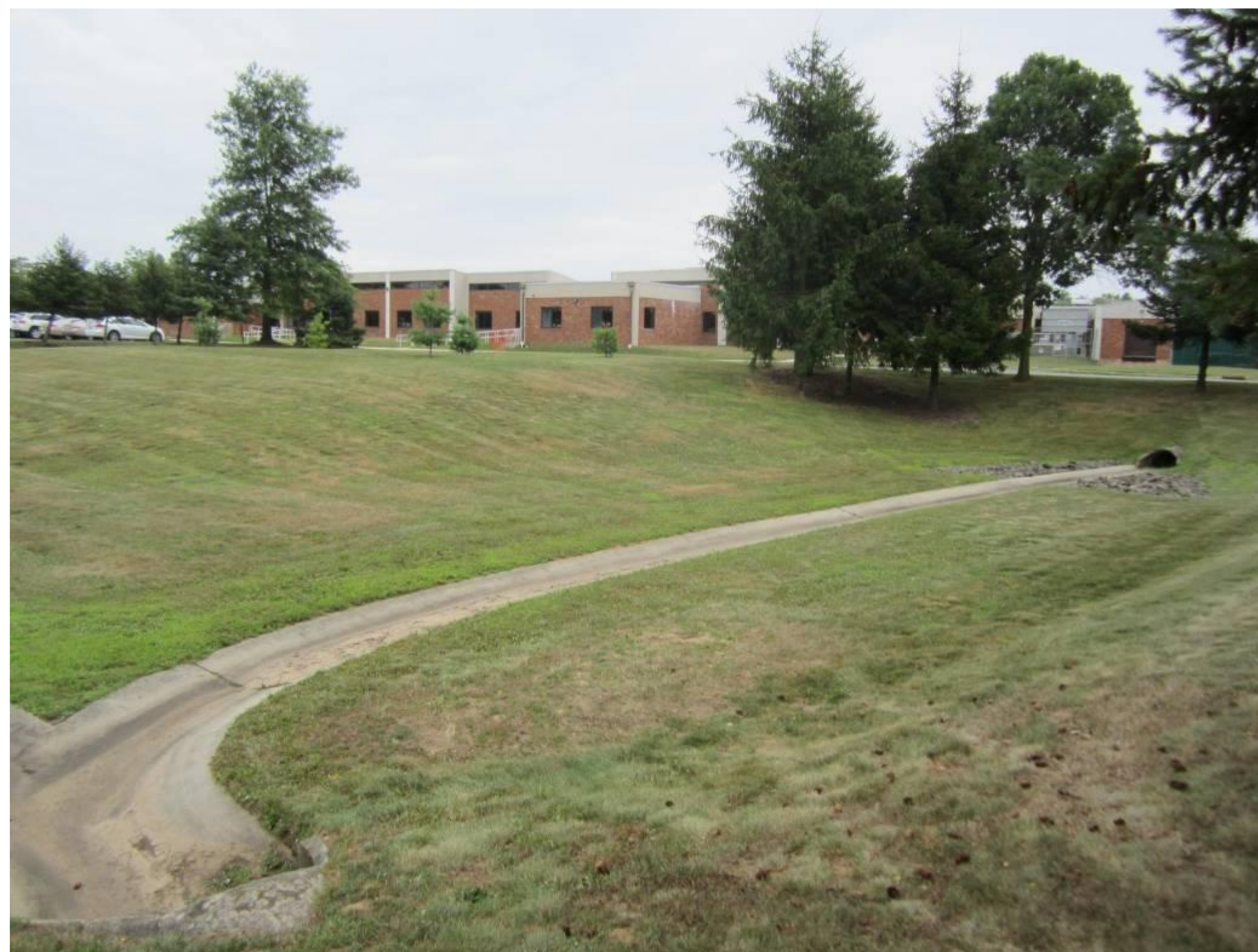
18" Diameter inlet and low flow
