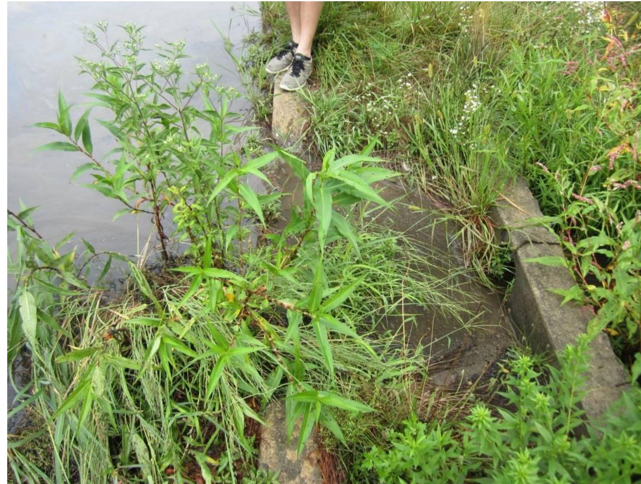
Inlet – curb cut
