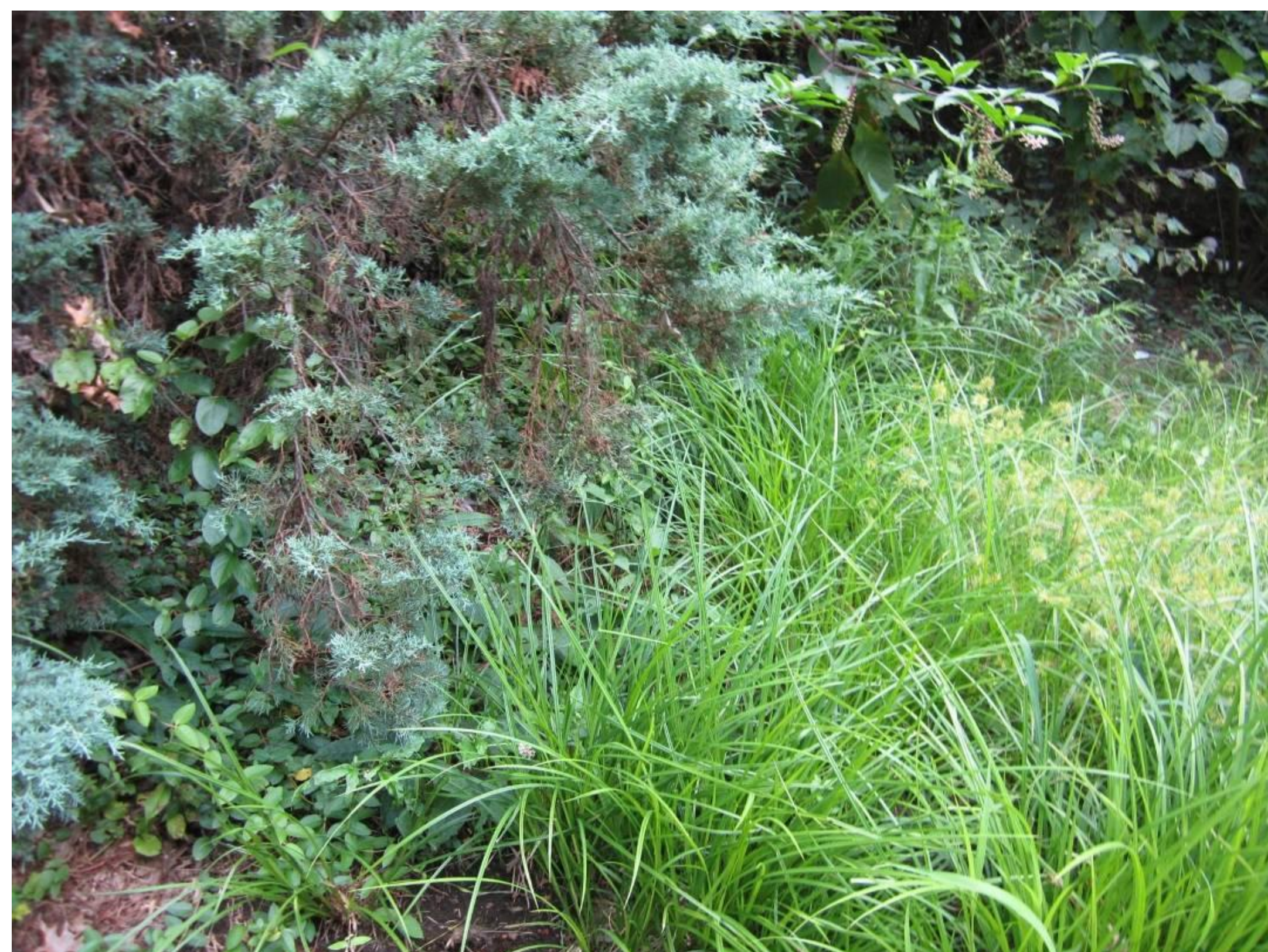
Excessive vegetative growth at inlet
