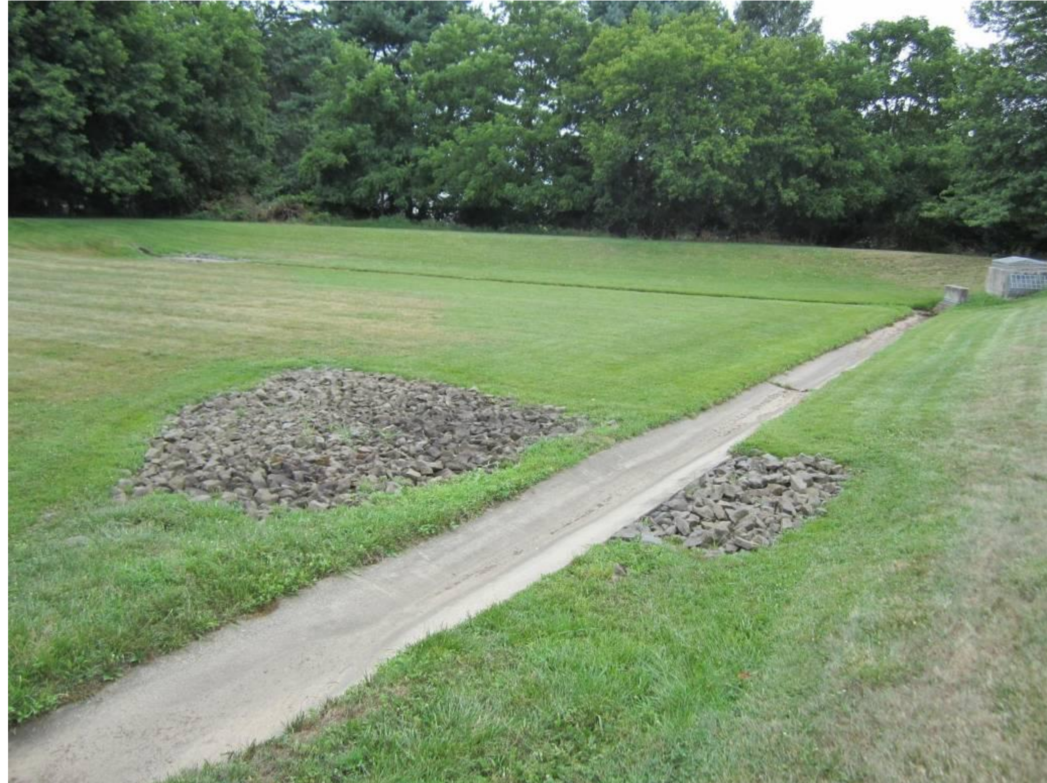
Low flow with rip rap protection
