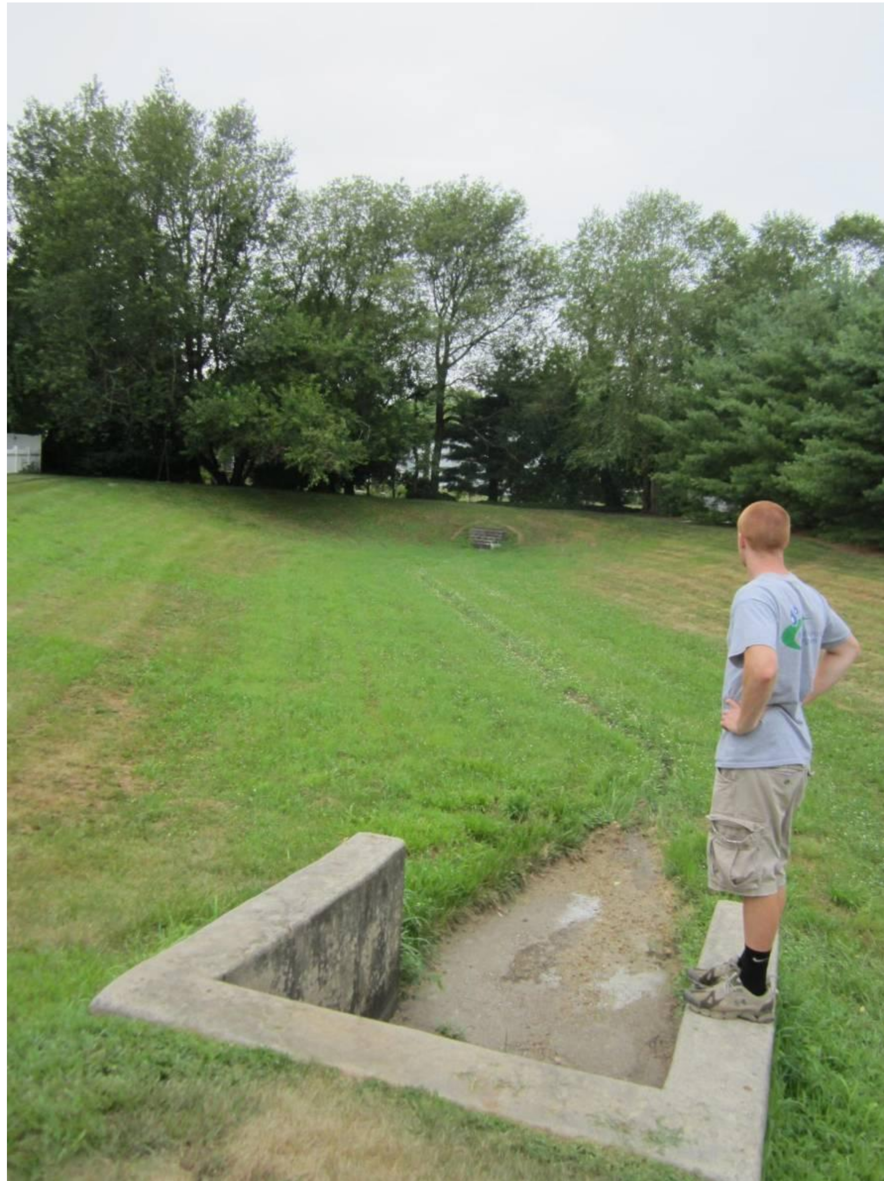
Basin bottom looking west
