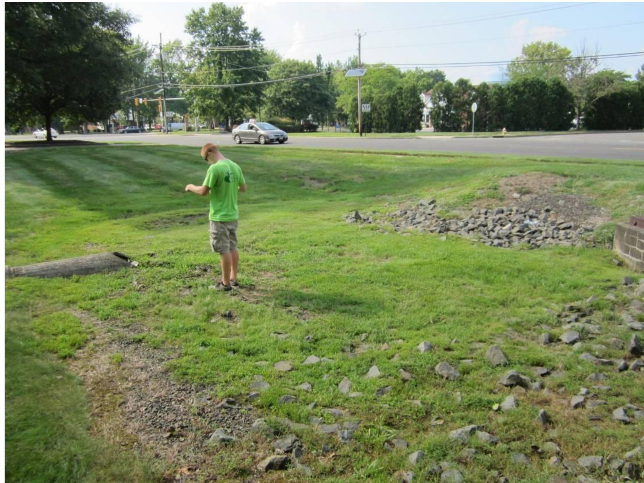
Basin bottom looking west
