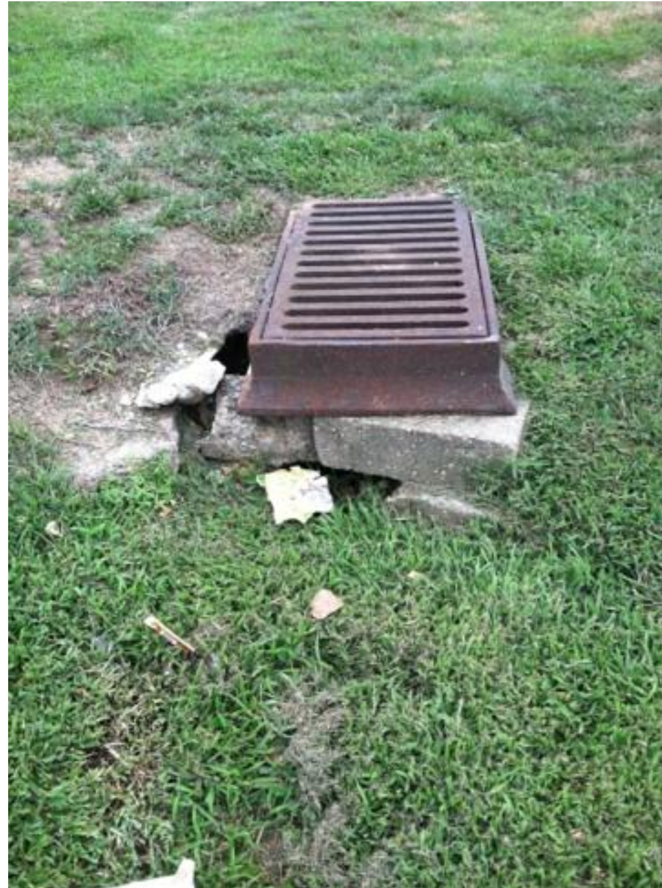
Damaged outlet
