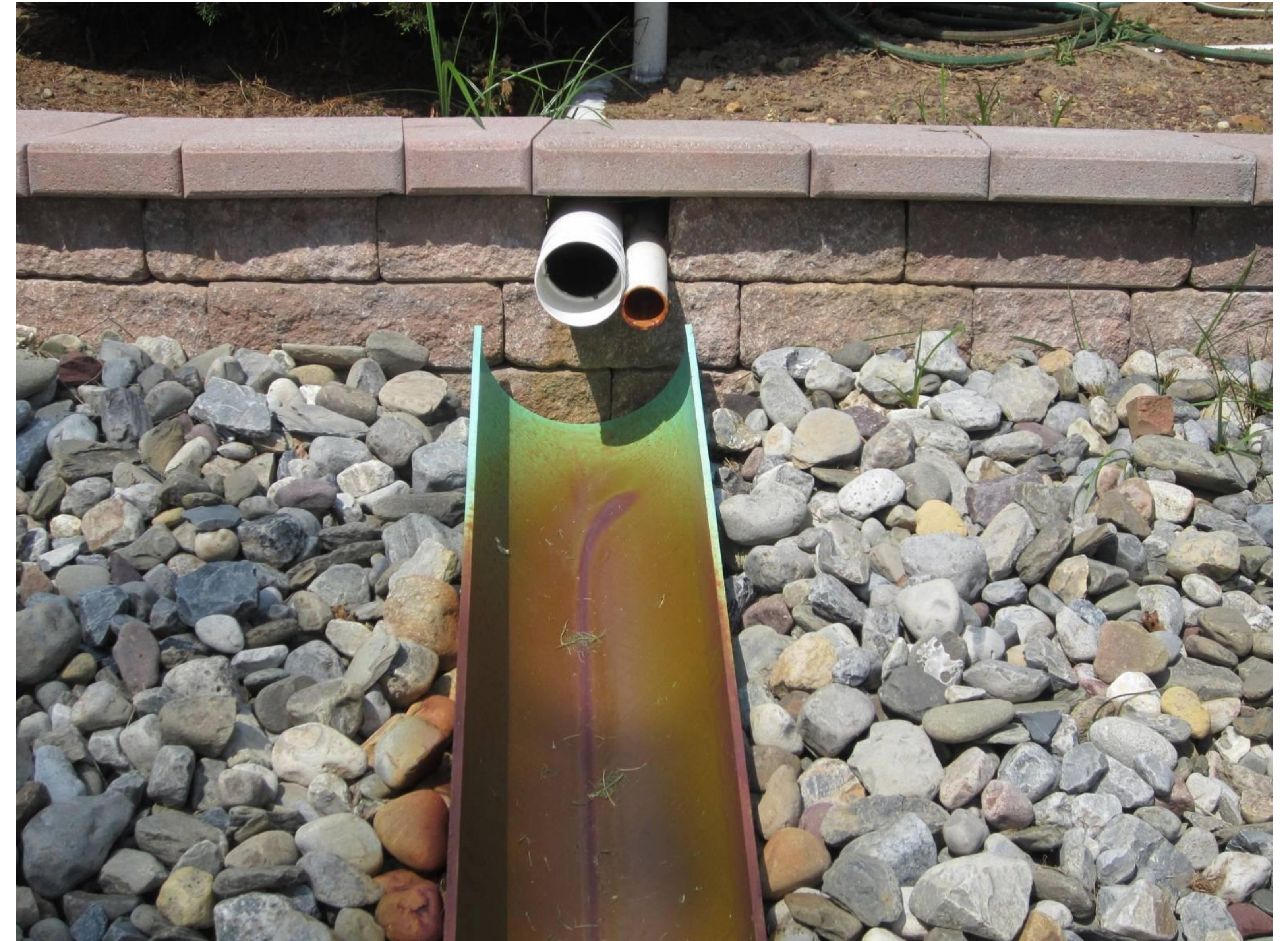
Pipe from rooftop run off
