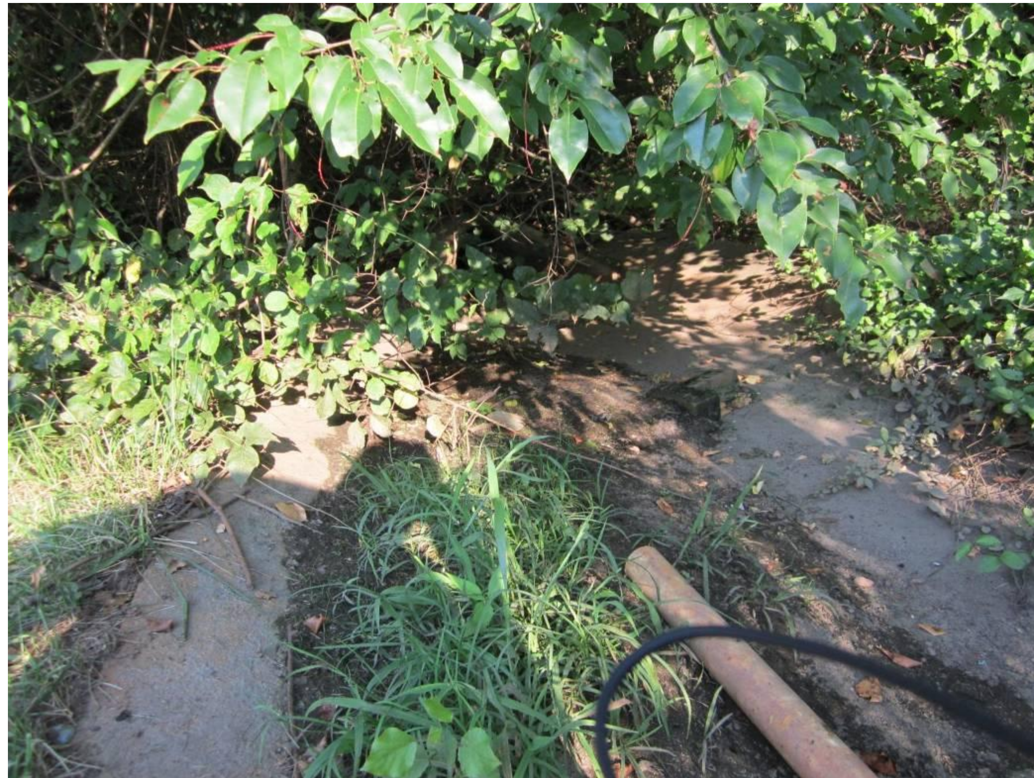
Inlet covered by plant growth
