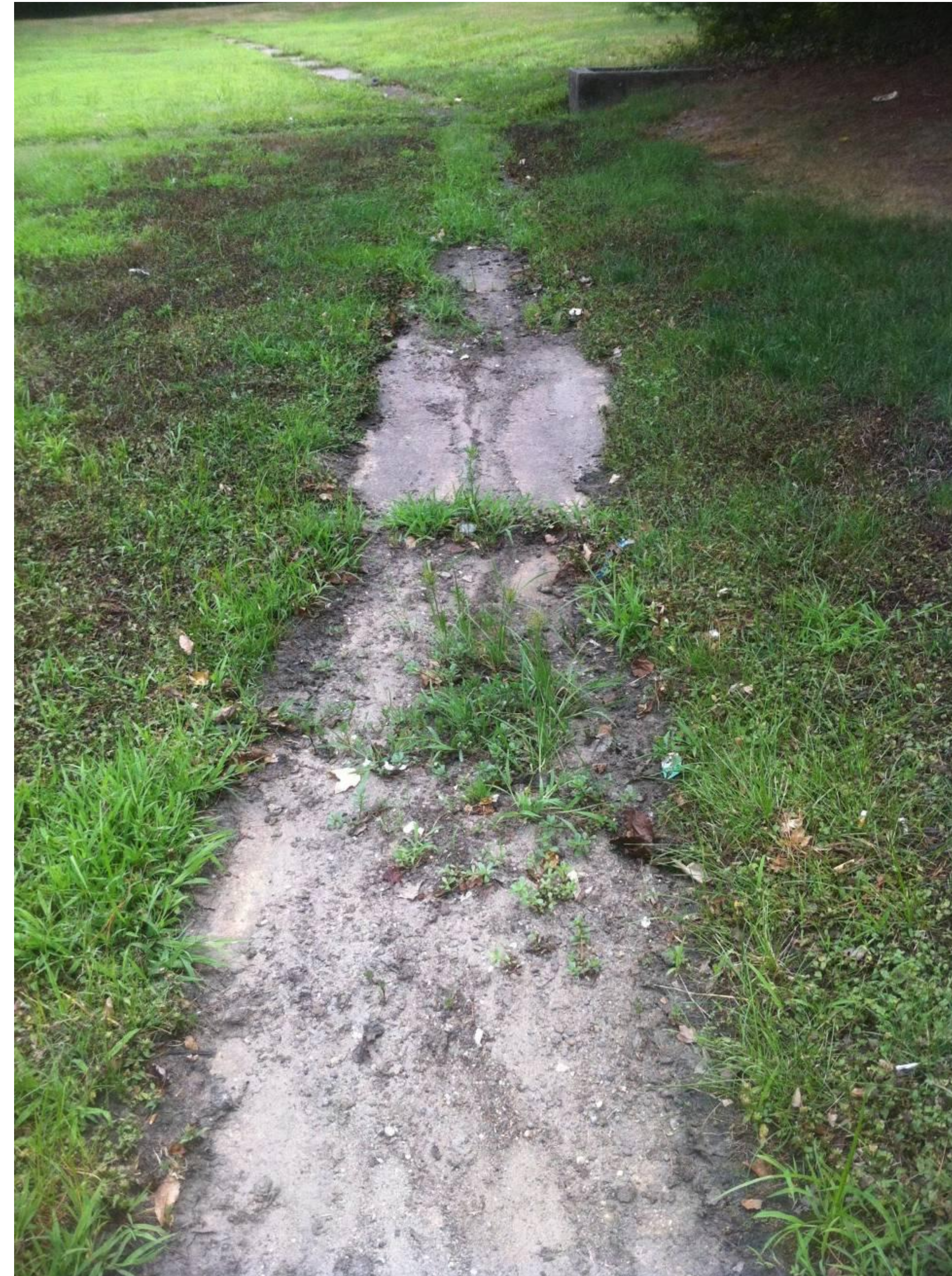
Sediment in low flow channel
