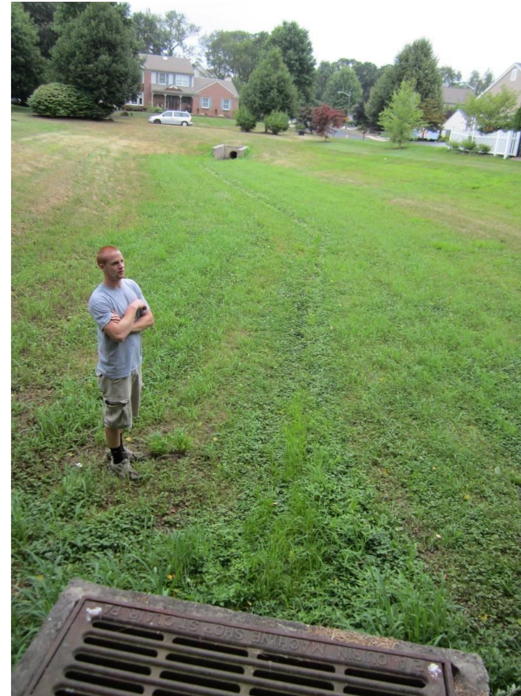
Basin bottom looking east
