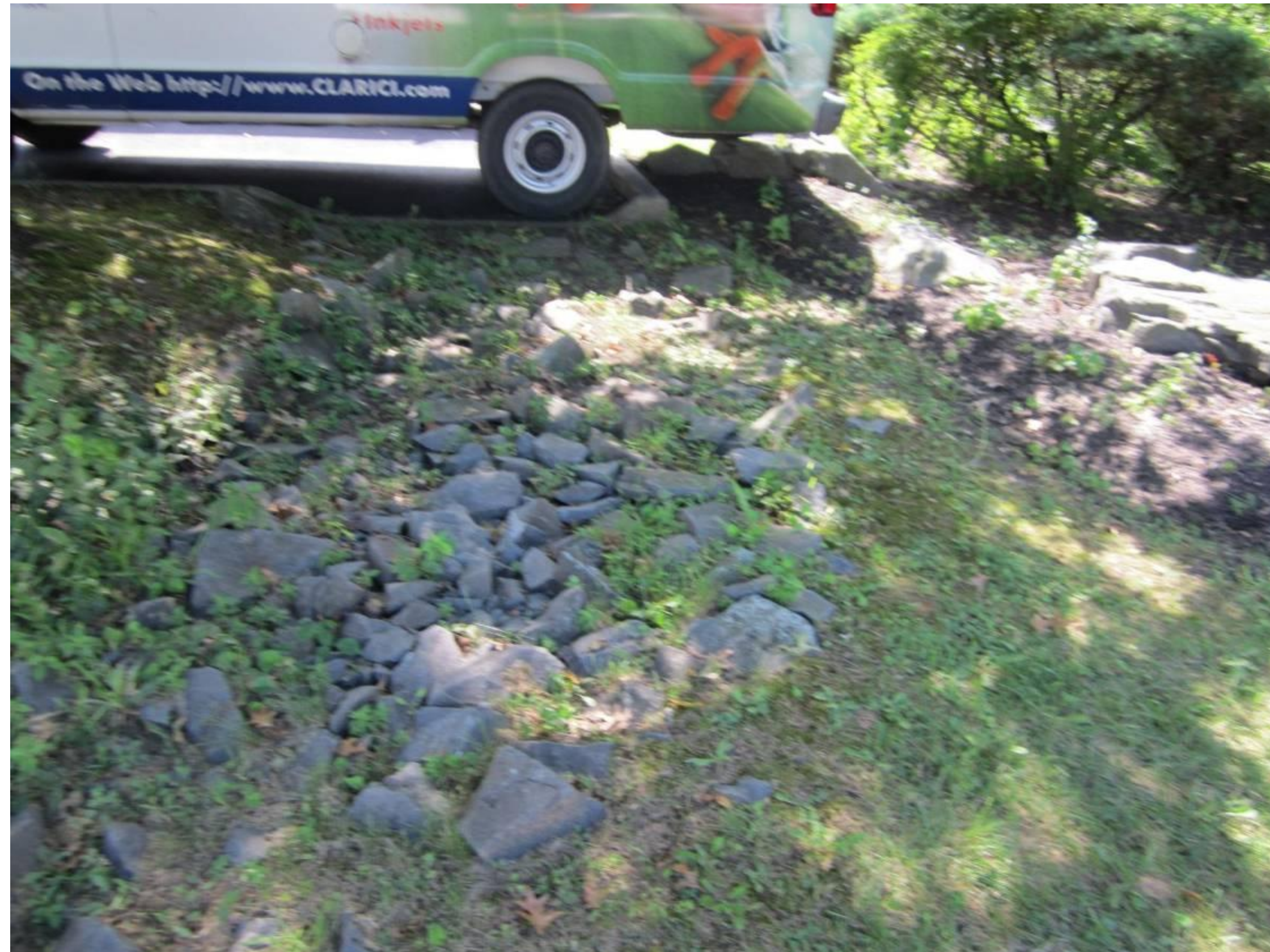
Curb cut inlet with rip rap protection
