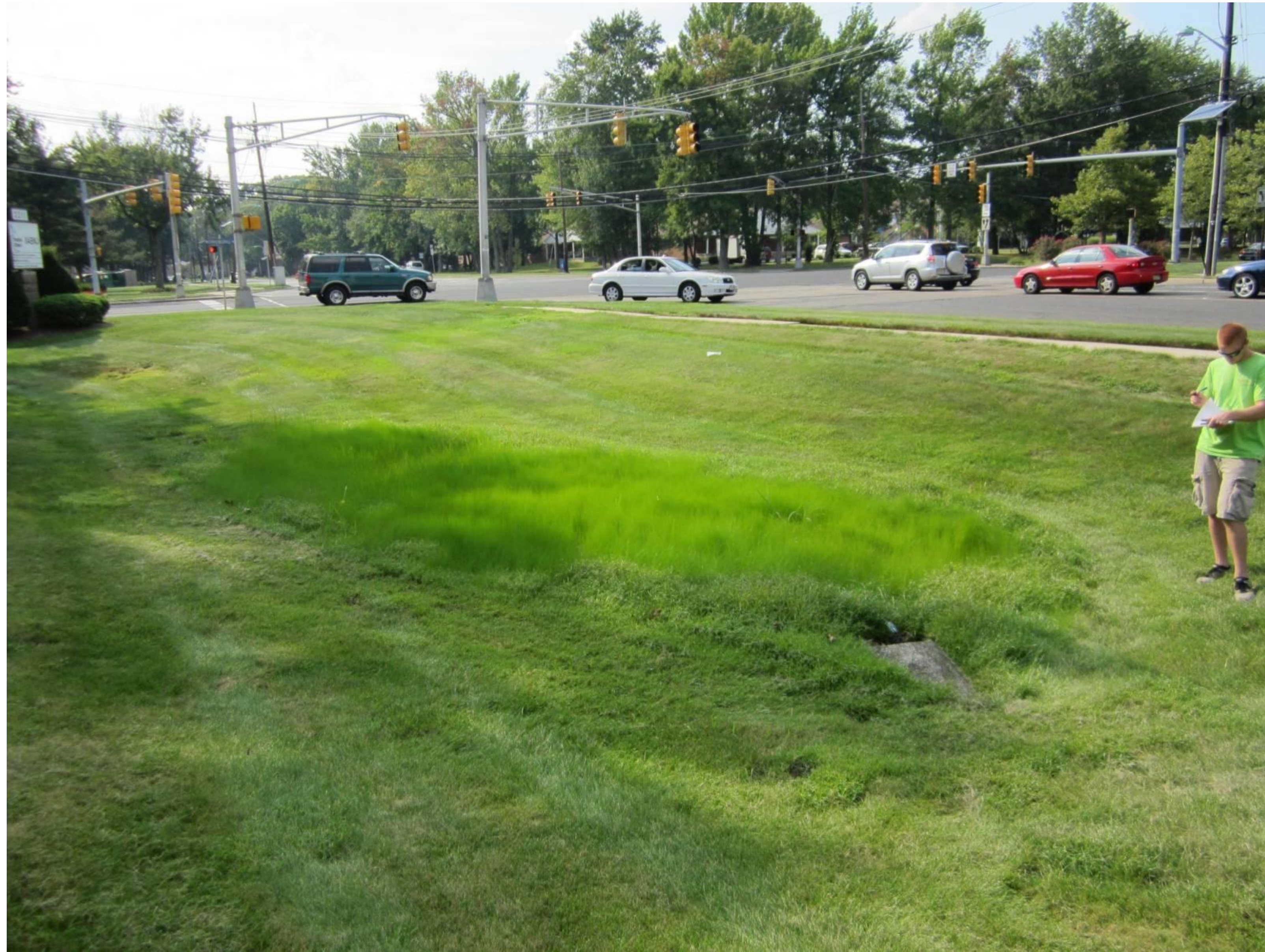
Basin bottom looking west
