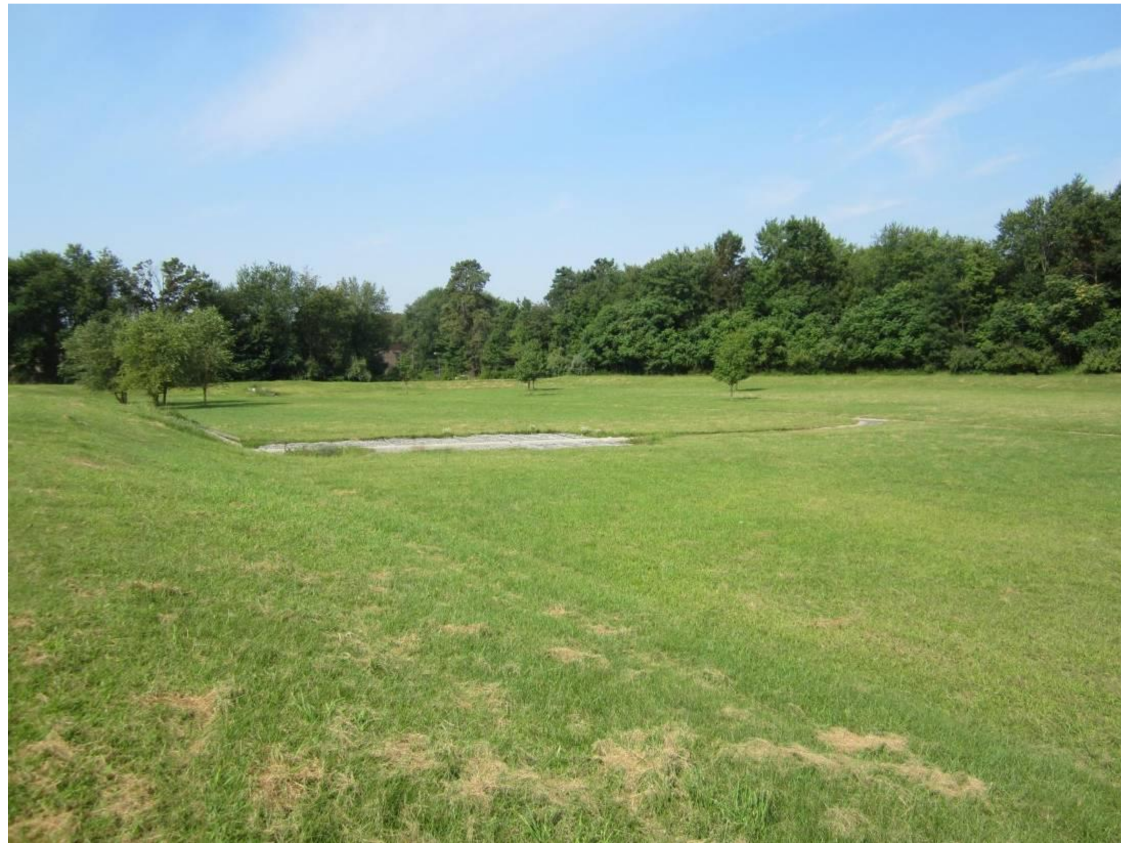
Basin bottom looking southwest
