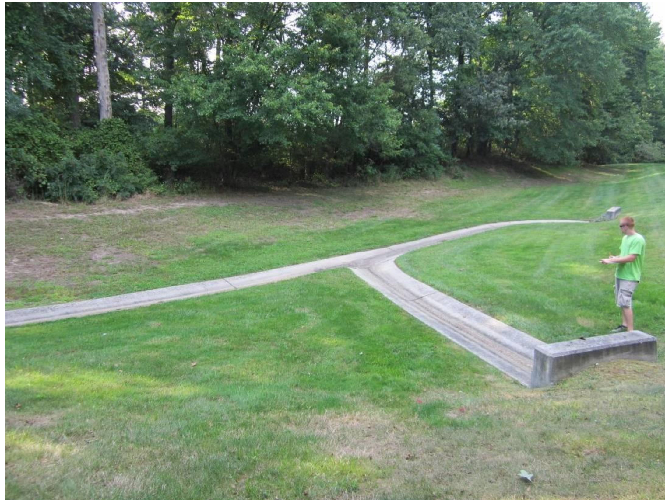
Basin bottom looking north
