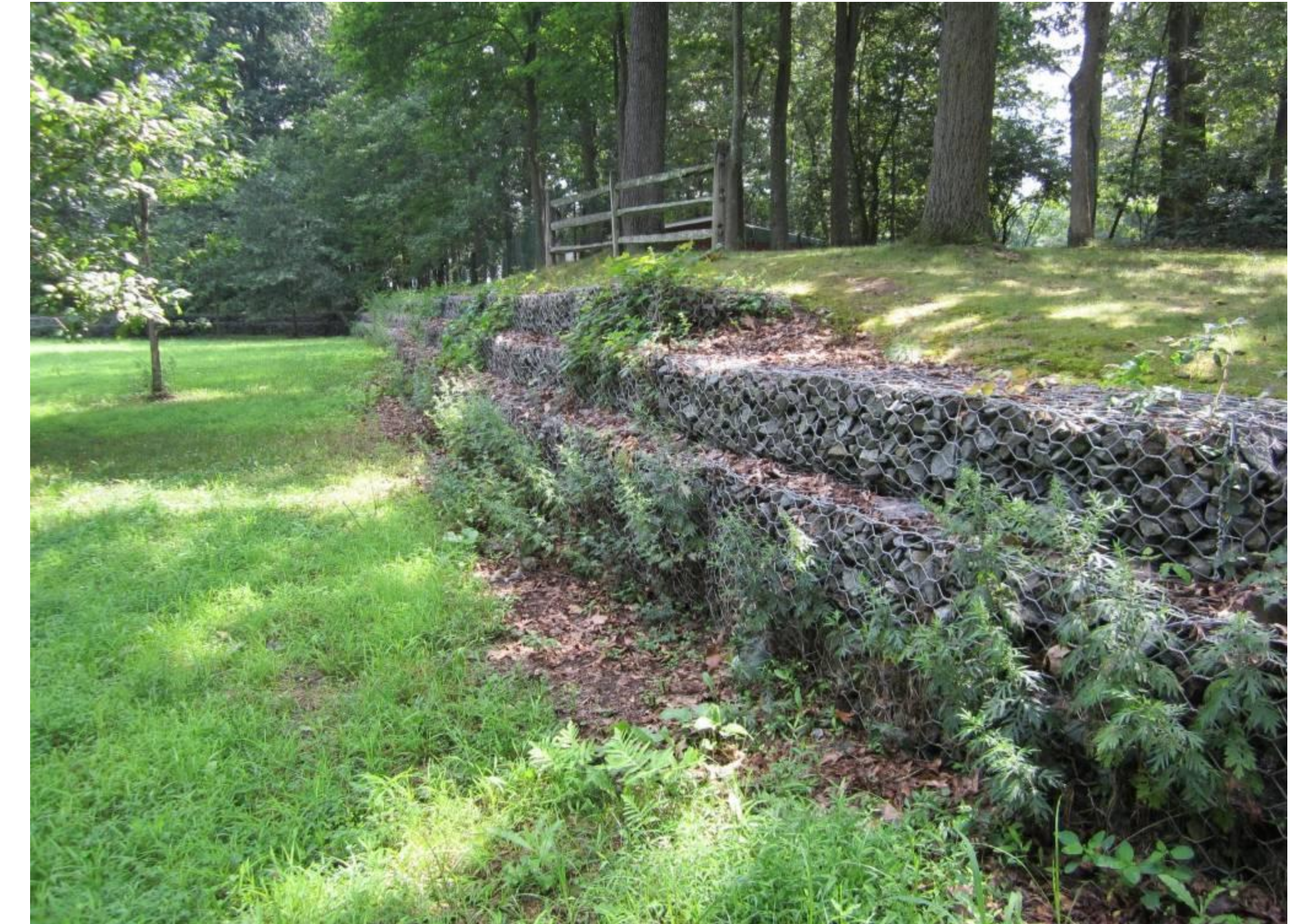
Gabion wall perimeter
