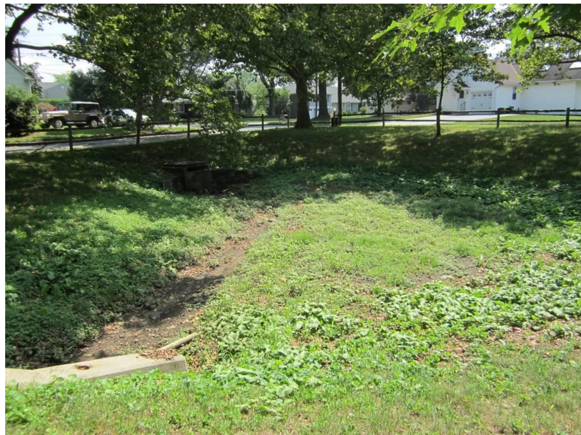
Basin bottom looking southeast
