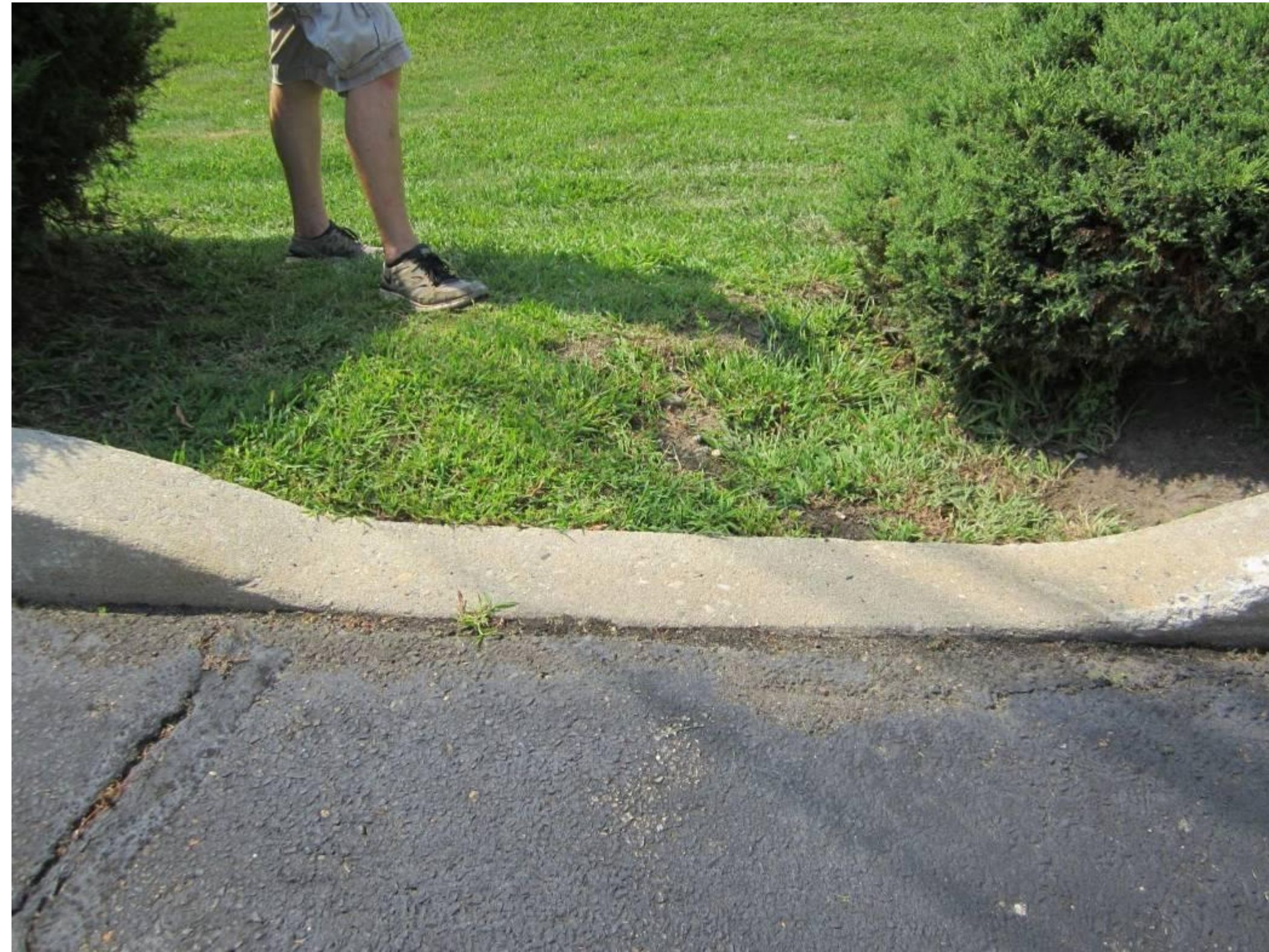
Curb cut inlet
