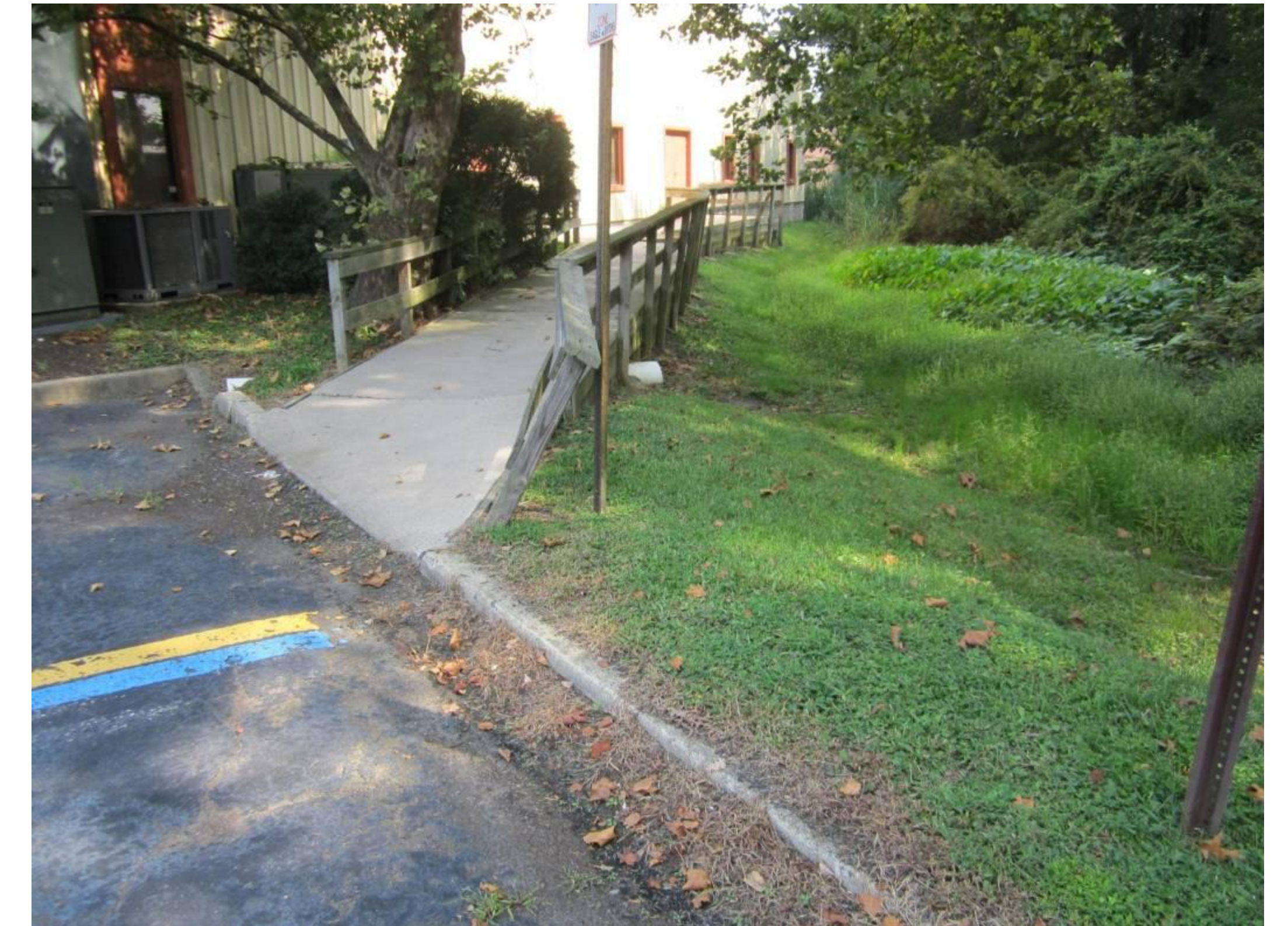
Basin bottom looking north
