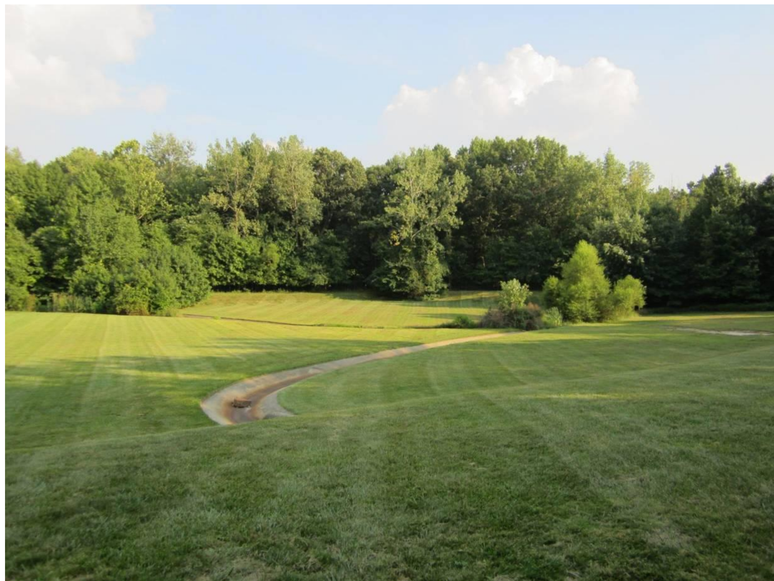
Basin bottom looking northwest
