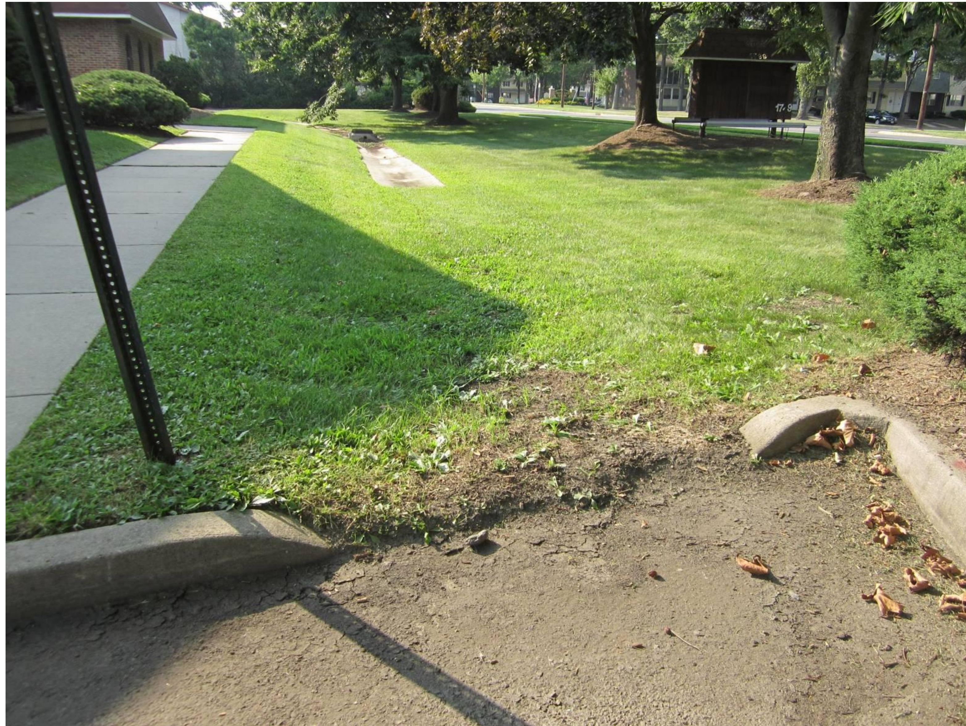
Inlet curb cut
